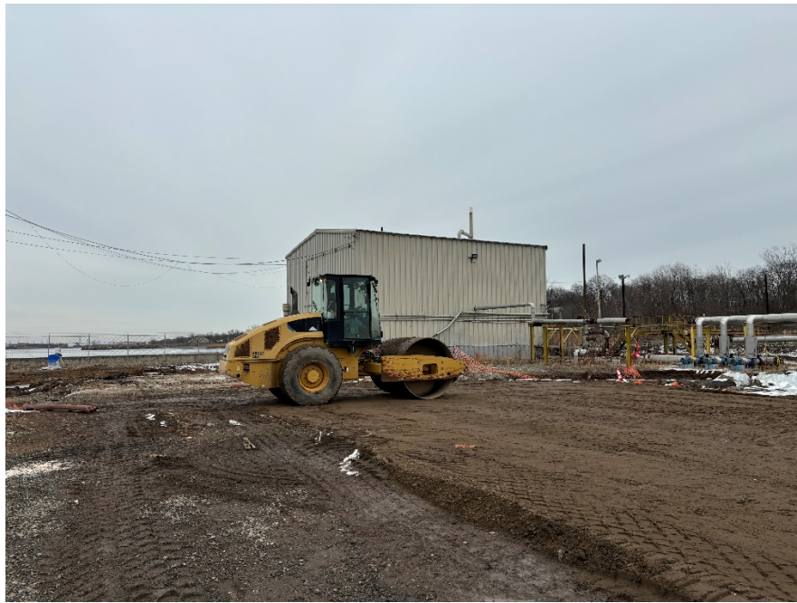
Photo 3: View of compaction at Excavation 5, IRM 1 Eastern Area, facing northeast.
