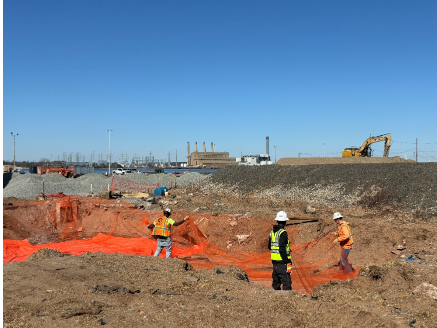
Photo 3: Placement of demarcation layer at Excavation 12B, IRM 1 Central Area, facing west.
