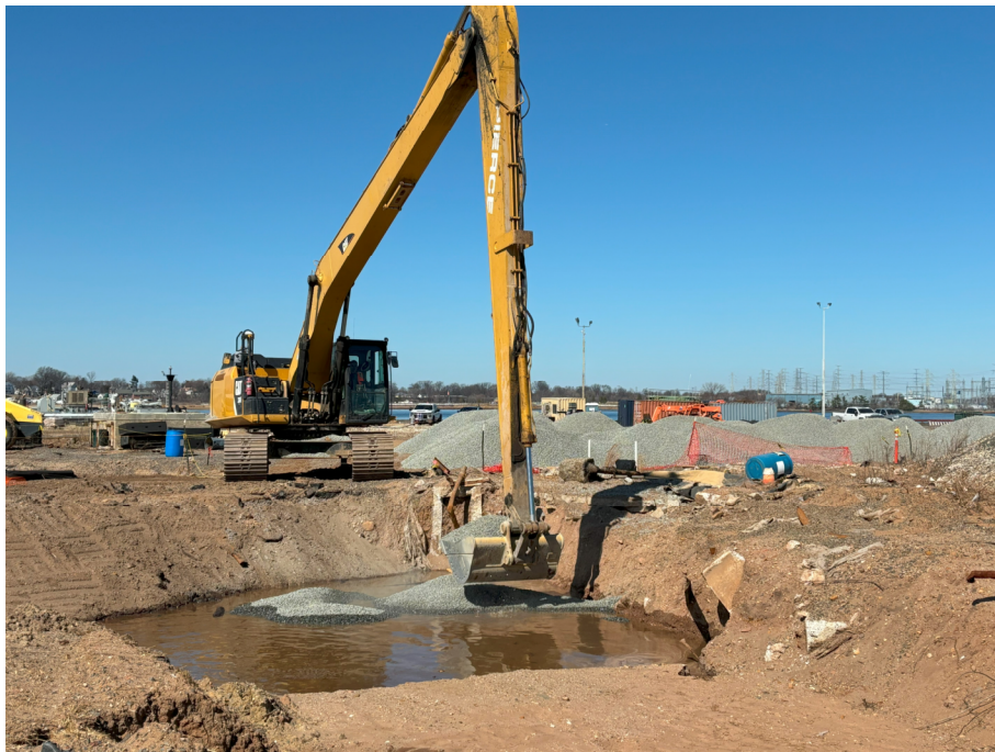
Photo 2: View of stone placement in Excavation 12B, IRM 1 Central Area, facing west.
