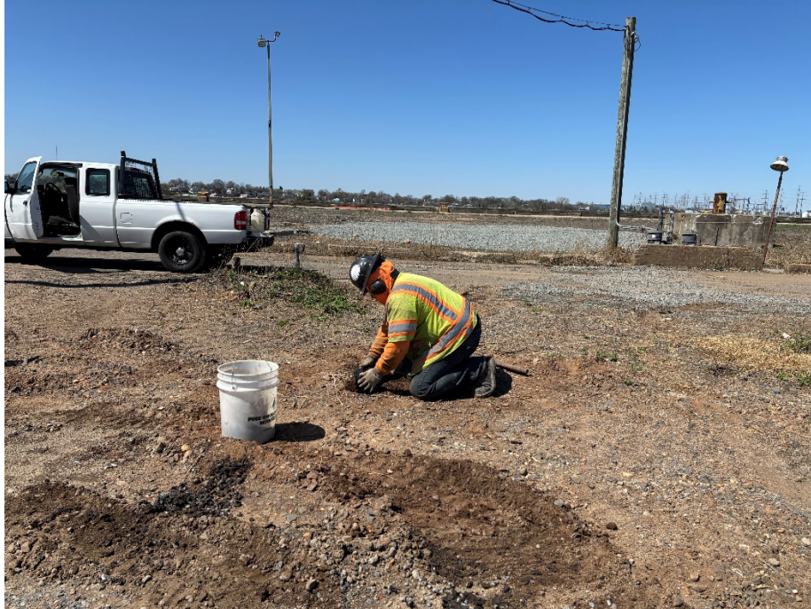
Photo 4: View of flush mount installation for MW-EX6, facing west.
