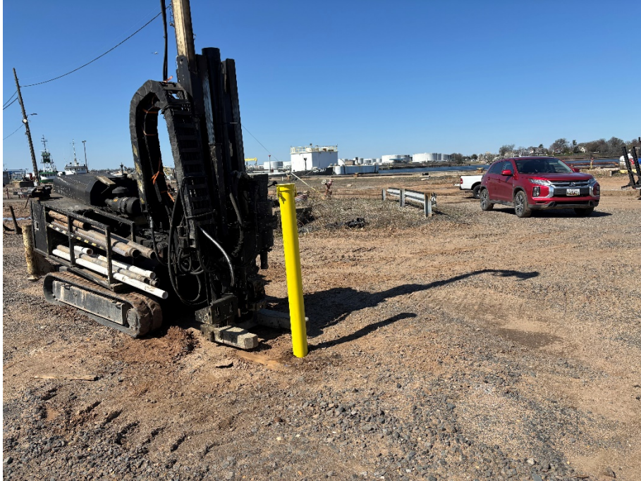
Photo 3: View of installation of stick-up monitoring well for MW-EX11, facing west.
