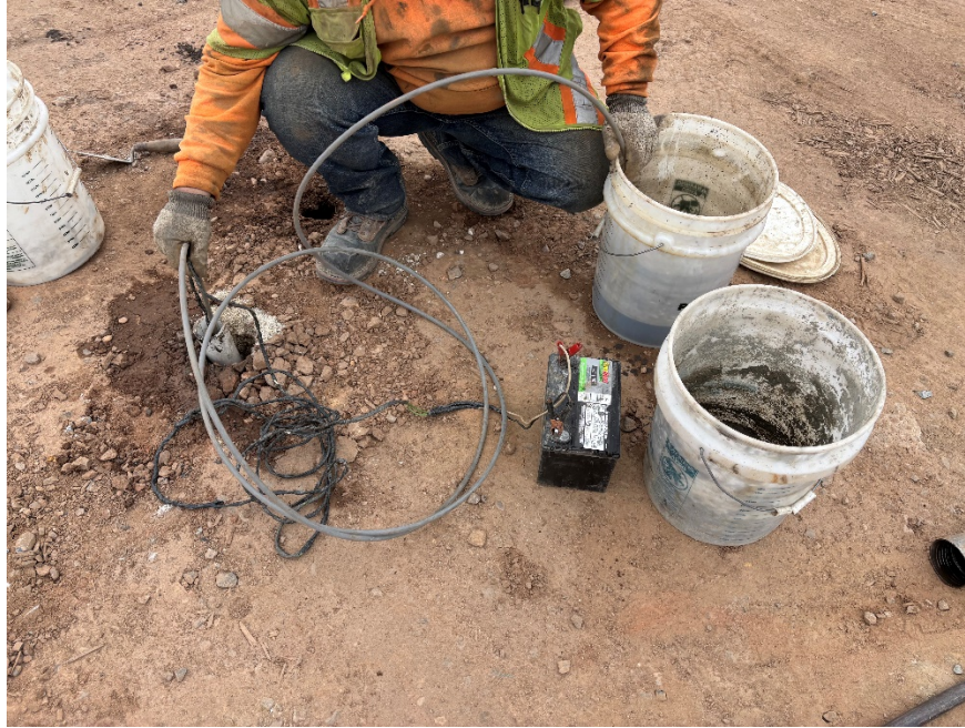
Photo 3: View of well development at MW-EX14, facing north
