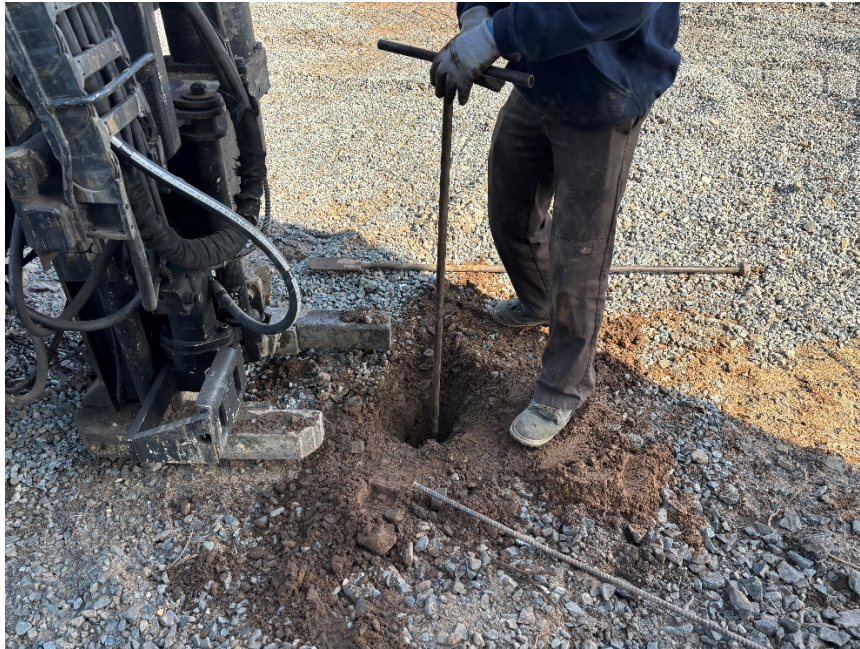
Photo 1: View of soft-digging at MW-EX4A prior to installation, facing south.
