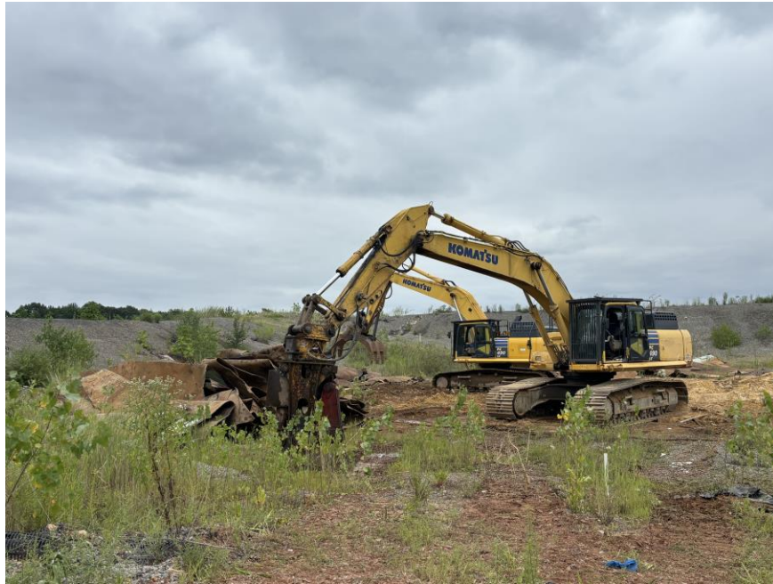
Photo 1: View of steel tank bottom demolition at AST 12, facing northeast.
