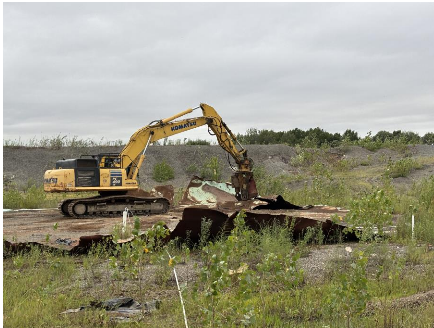
Photo 2: Alternate view of steel tank bottom demolition at AST 12, facing east.
