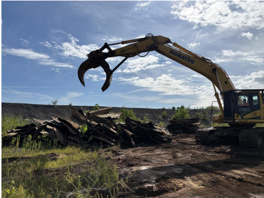
Photo 2: View of steel C&D debris stockpile at AST-12, facing northeast.
