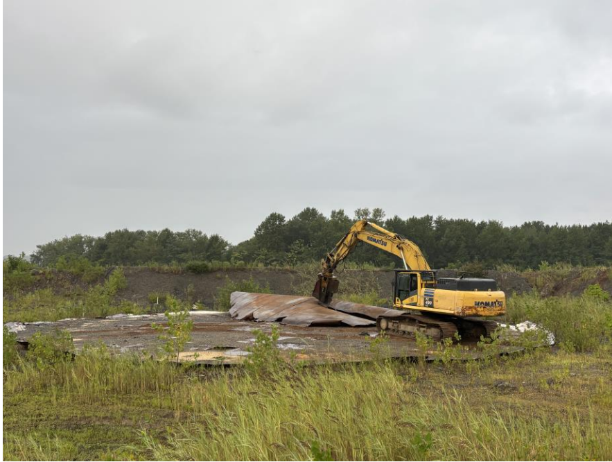
Photo 1: View of steel tank bottom demolition at AST-11, facing west.
