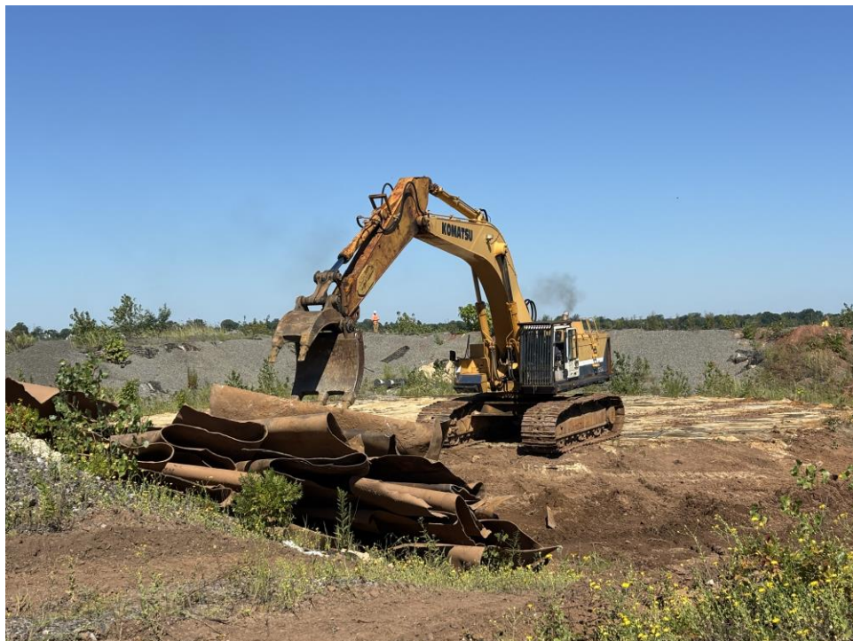
Photo 2: View of steel C&D debris stockpile at AST-9, facing west.
