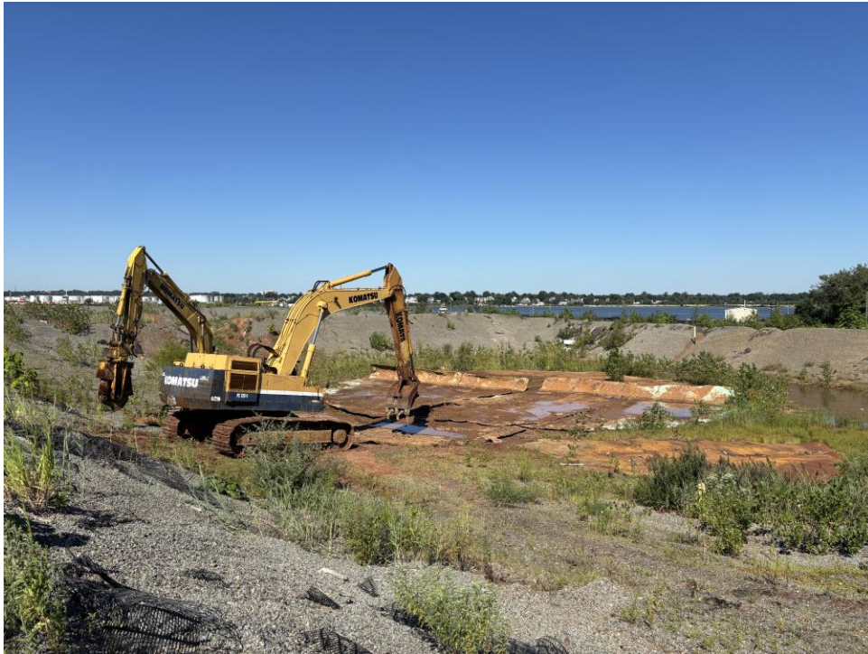
Photo 1: View of steel tank bottoms demolition at AST-10, facing west.
