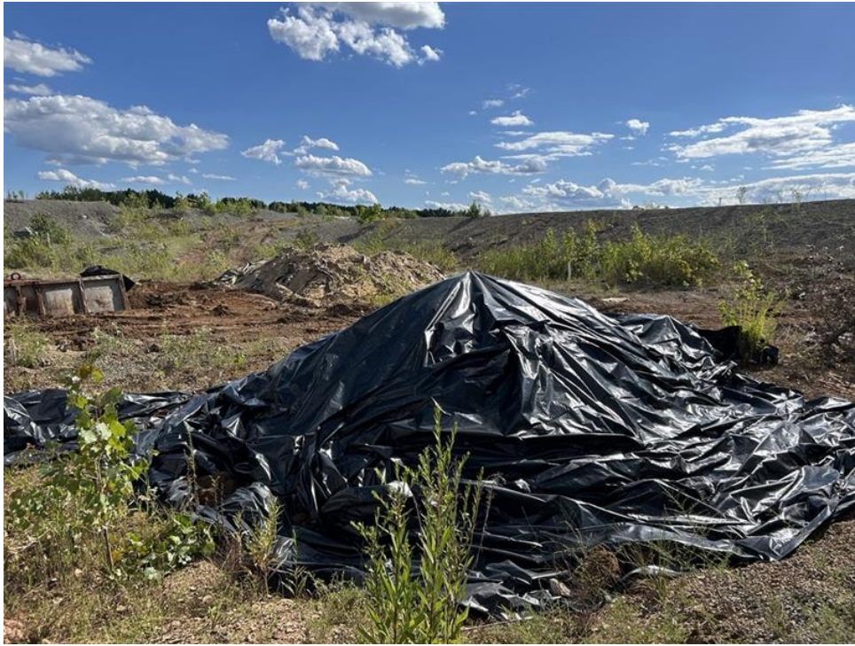
Photo 1: View of ISS overburden soil stockpile, facing west.
