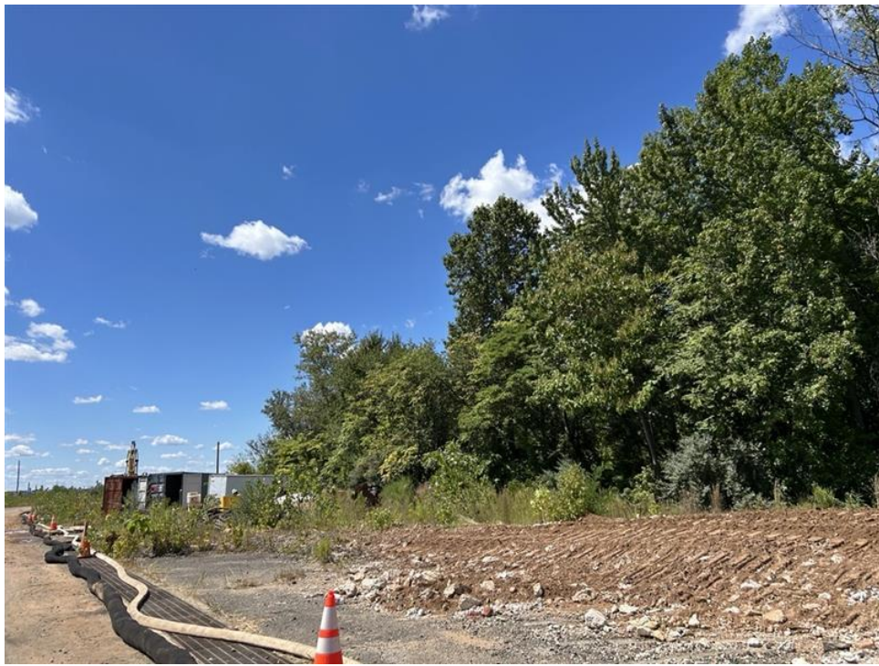
Photo 2: View of Entact equipment staging area for ISS pilot test, facing northeast.
