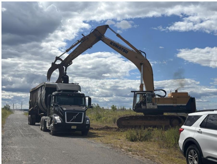
Photo 2: View of steel C&D debris being loaded for off-site disposal, facing south.
