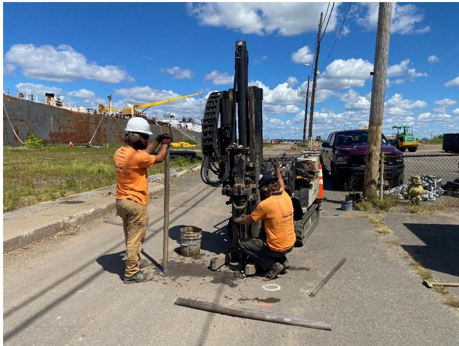
Photo 2: View of Lakewood soil boring installation activities along PRB wall segment 3, facing north.
