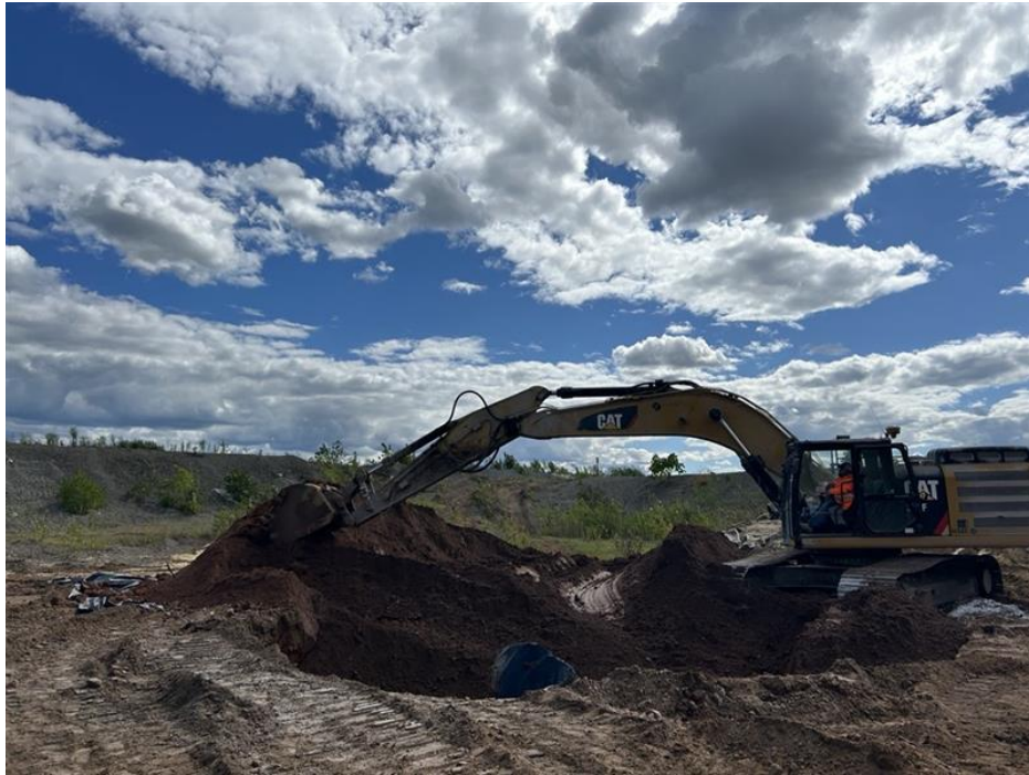
Photo 1: View of Entact dry mixing ISS reagents and soil in cell 1A, facing northeast.
