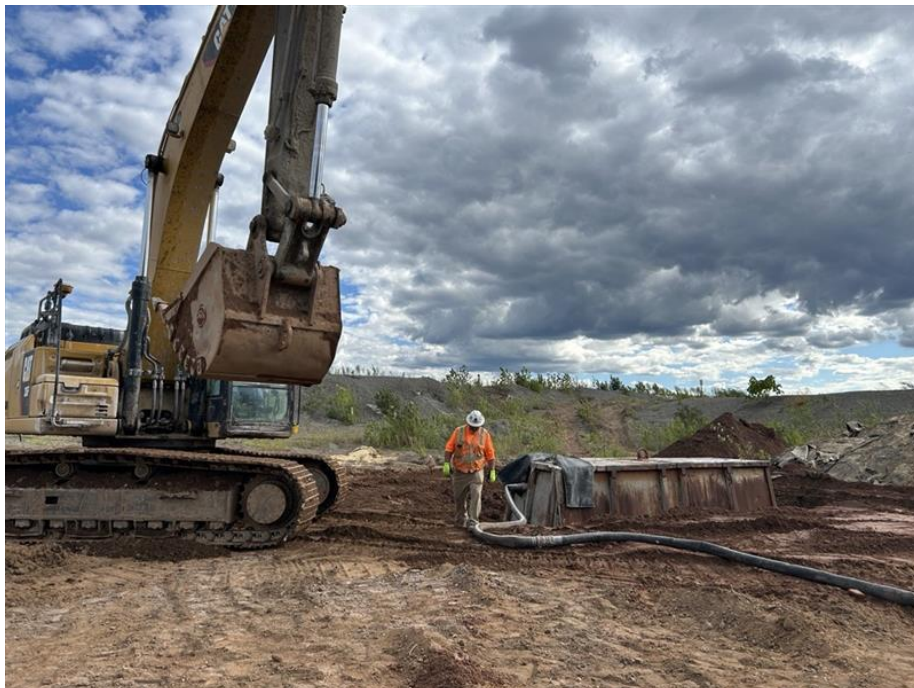
Photo 2: View of Entact pumping ISS reagents into containment box for dry mixing in cell 1A, facing northeast.
