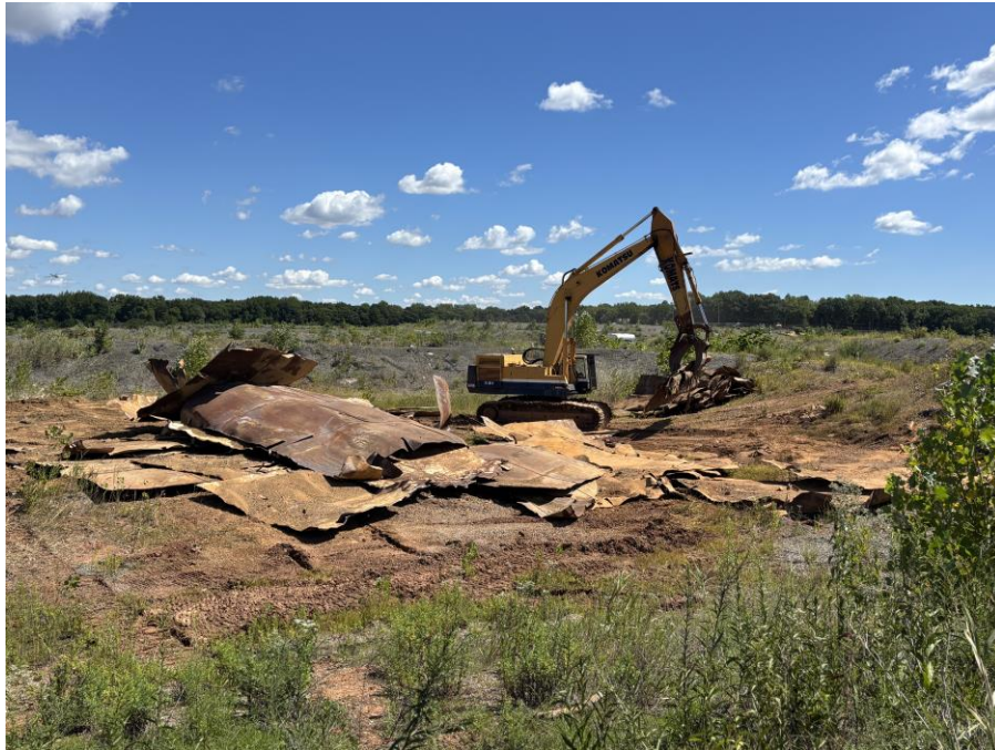
Photo 1: View of steel tank bottoms demolition at AST-8, facing northeast.
