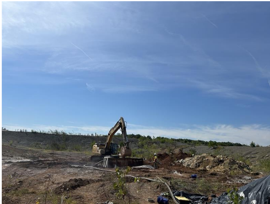
Photo 2: View of Entact pumping ISS reagents into containment box for dry mixing in cell 3A, facing south.
