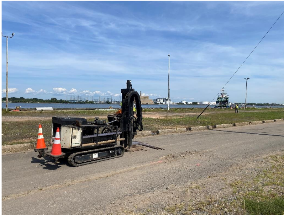
Photo 1: View of Lakewood soil boring installation activities along PRB wall segment 3, facing northwest.
