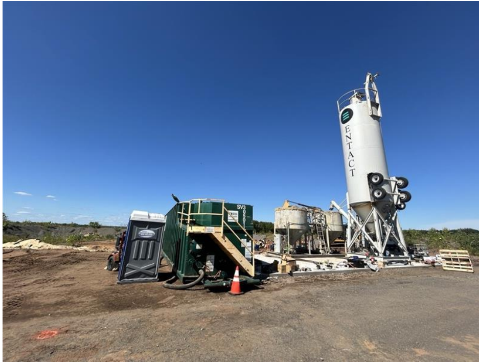
Photo 3: View of water storage frac tank staging adjacent to vertical reagent silos and dual grout mixing tanks, facing northwest.
