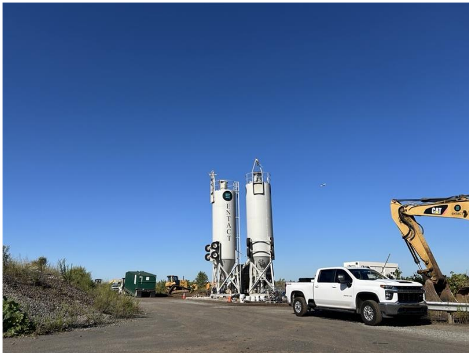
Photo 4: Alternate view of water storage frac tank staging adjacent to vertical reagent silos and dual grout mixing tanks, facing west.
