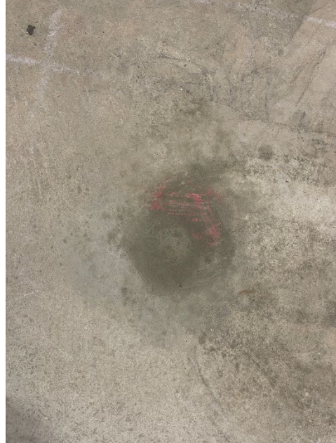
Photo 4: Sealed drilled area after hitting GW
