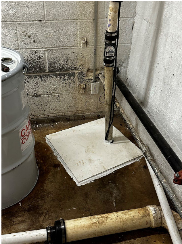
Photo 5: Secondary sump lid sealed
