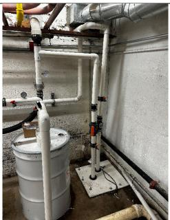
Photo 3: Final set up of the SVE system
