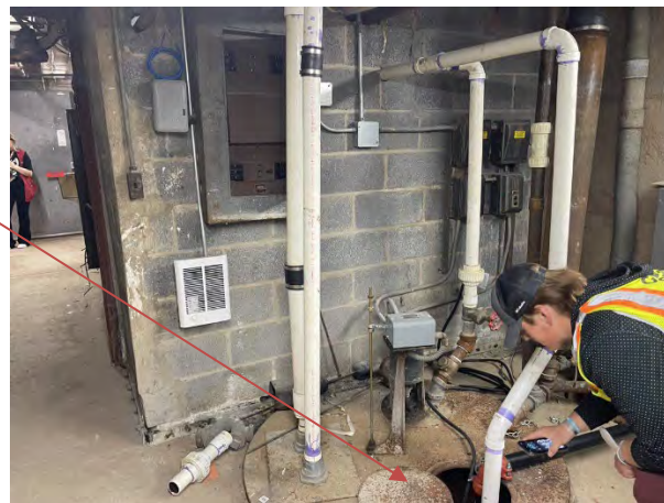
Photo 2: West Room: Piping from the large north sump into the LPGAC vessels have been valved closed. Therefore, water extracted from the sump bypasses the LPGAC and flows untreated into the sewer system
