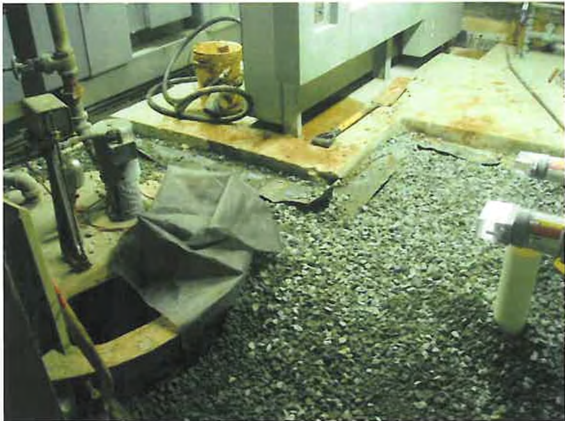
EQUIPMENT ROOM BACKFILLED, NOTE VERTICAL PIPE
