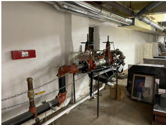
Photo 5: Temporary drain that was installed under the sprinkler system that drains into the second north sump pit
