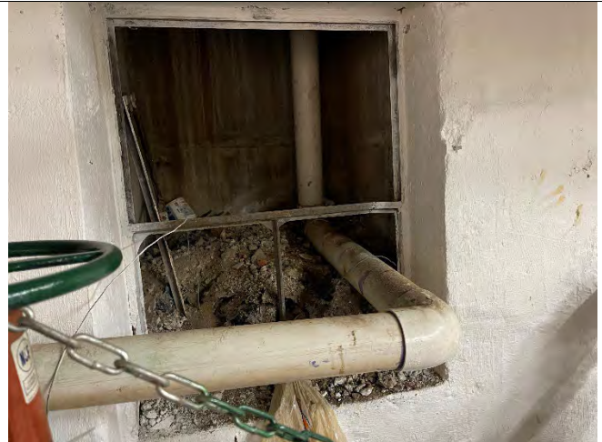
Photo 6: SVE exhaust piping to roof.
