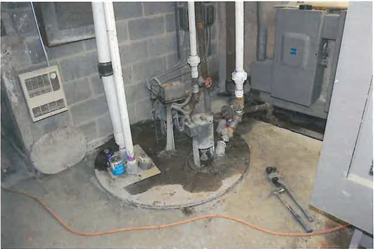
LARGE SUMP PIT WITH NEW PLUMBING
