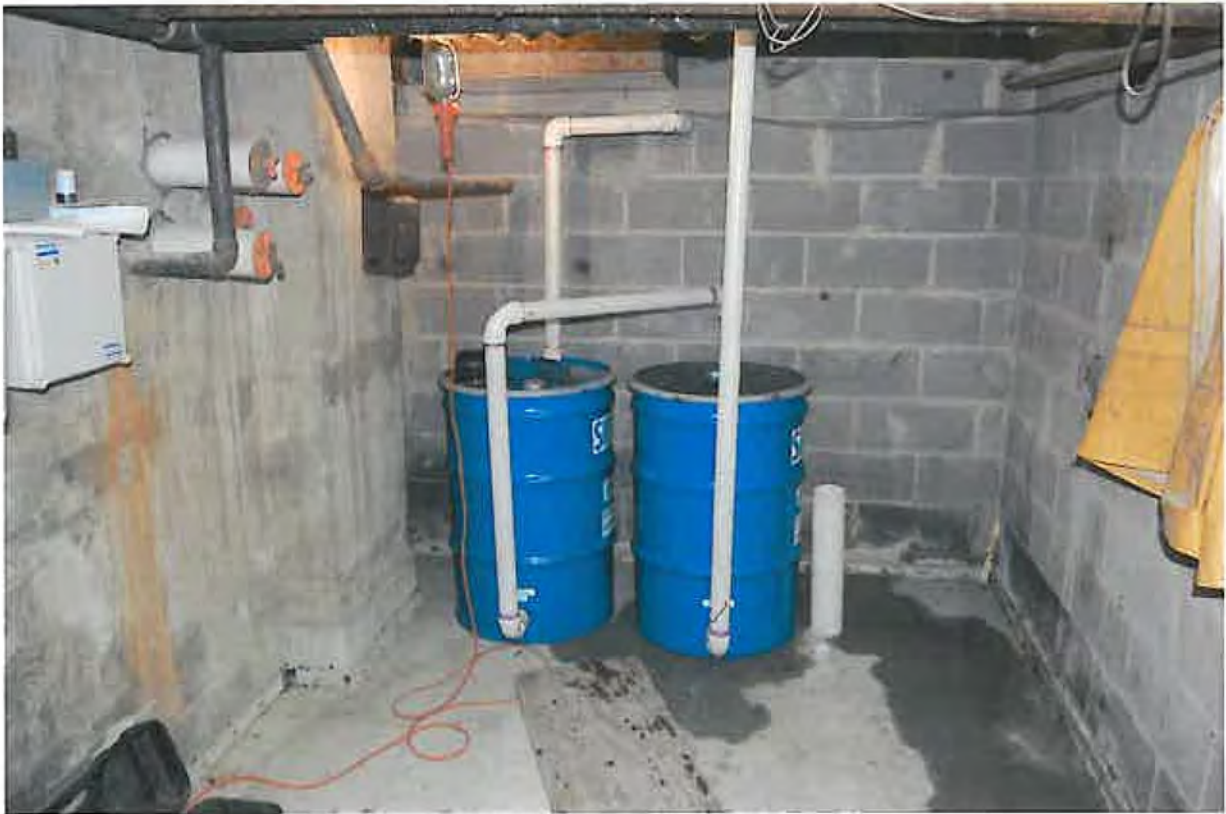
TWO LIQUID-PHASE CARBON FILTERS IN SERIES
