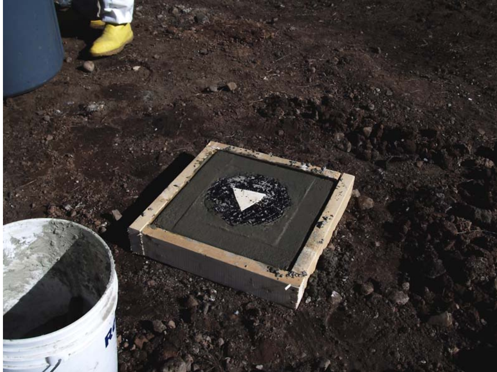
Photograph 6. 8 October 2010. Completion of well PO-1.
