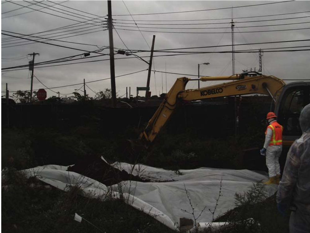
Photograph 1. 4 October 2010. Backhoe excavating Test Pit ZA-1.
