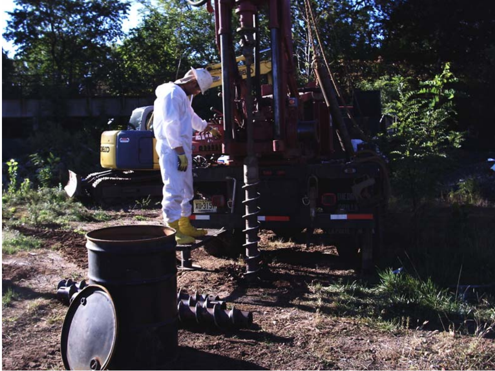
Photograph 5. 7 October 2010. Drilling well PO-2.
