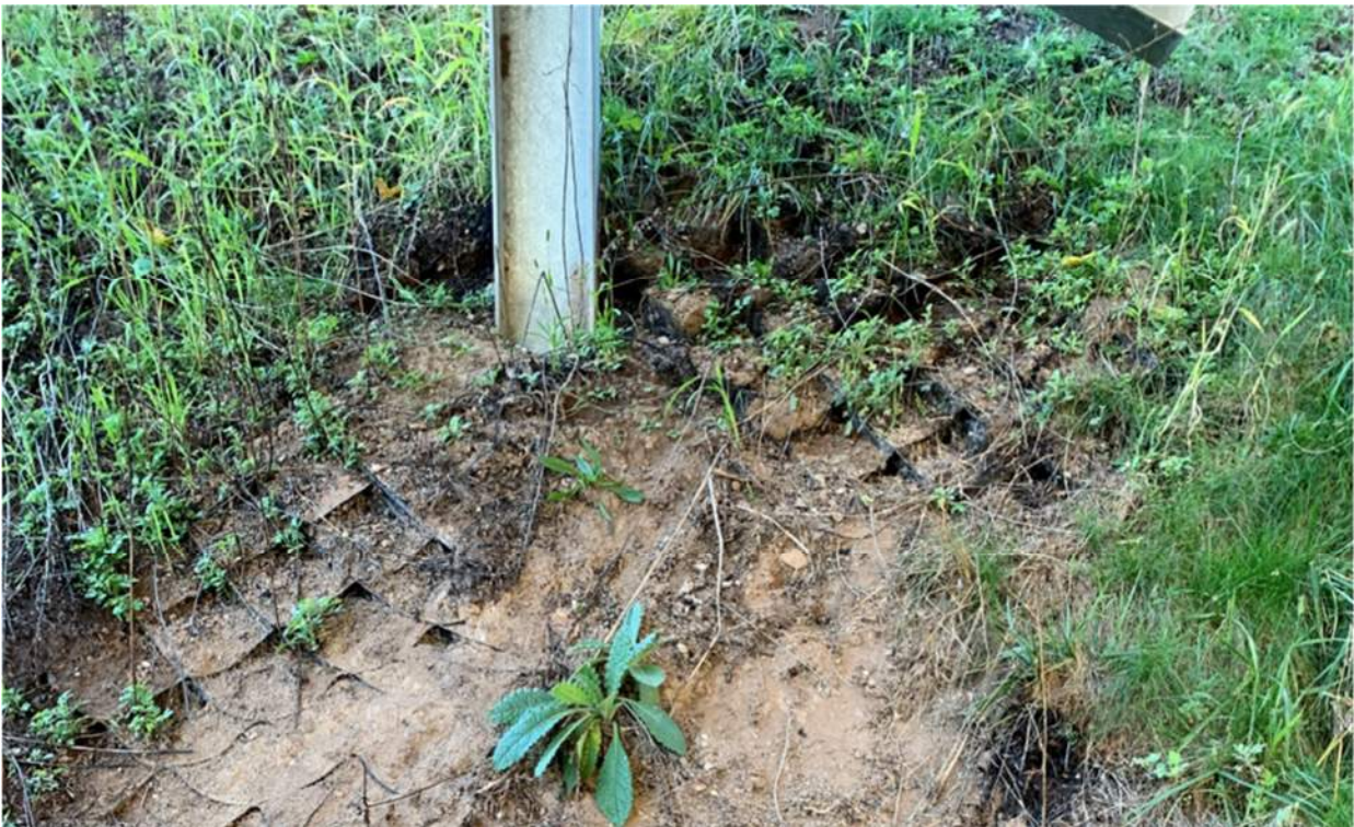
Photo 8: November 14, 2022 - New Fire Range – Soil Erosion on Inside of Berm
