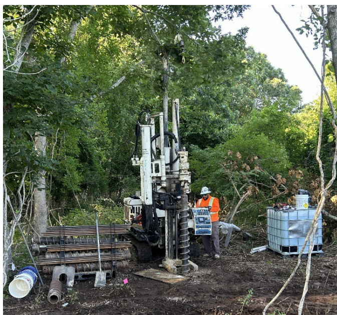
Figure 2: Monitoring well installation
