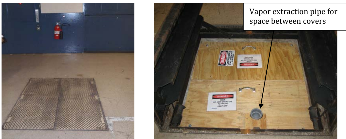
Exhibit 5.4 – Manhole No. 30. Double-door cover (left) and internal cover (right).
