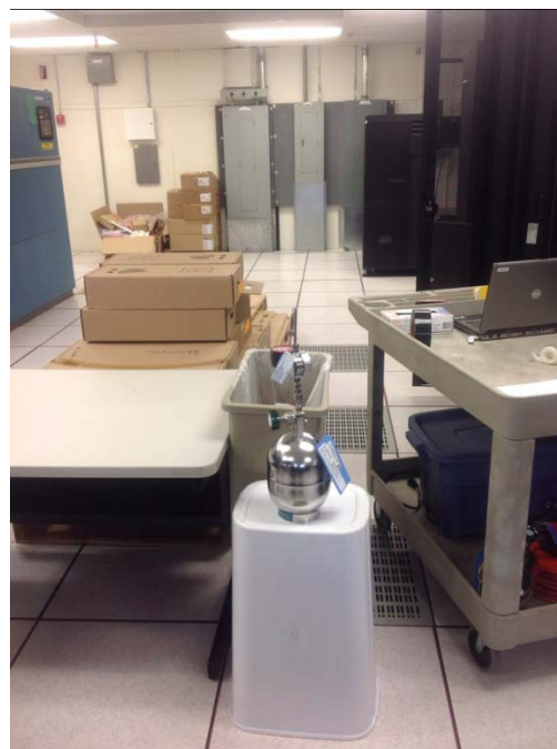
Photo #2: Sample IA1012, located in SAIL Lab (server room).
