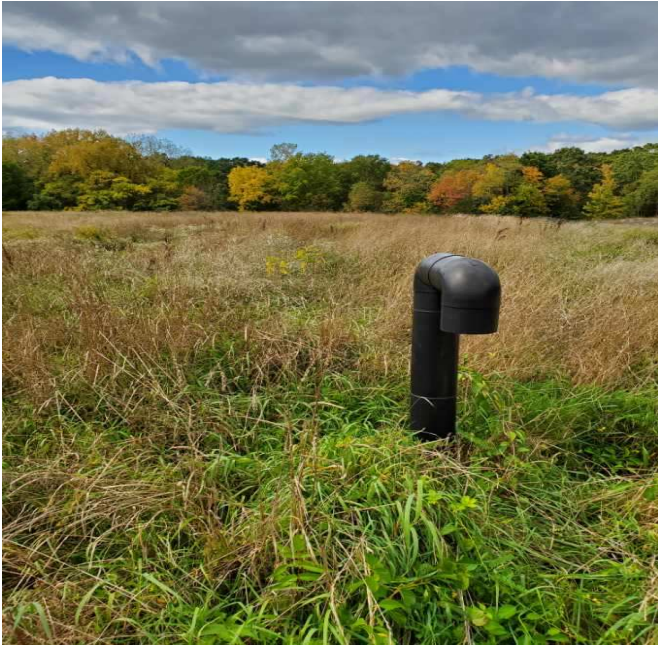
Photo 9: Looking south near north gate on the north portion of landfill. View of gas vent and landfill cap.
