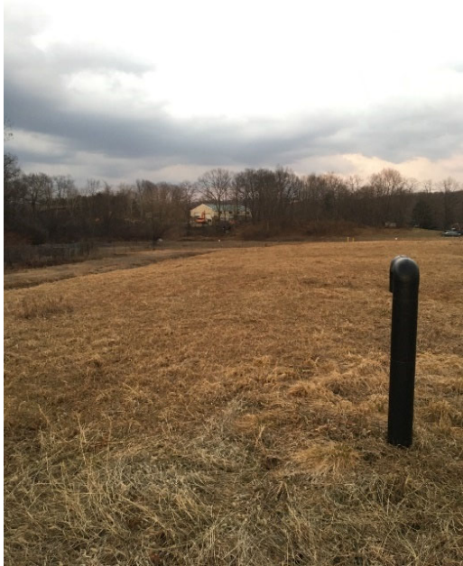
Photo 9: Looking east near north gate on north portion of landfill. View of gas vent and eastern portion of landfill cap.
