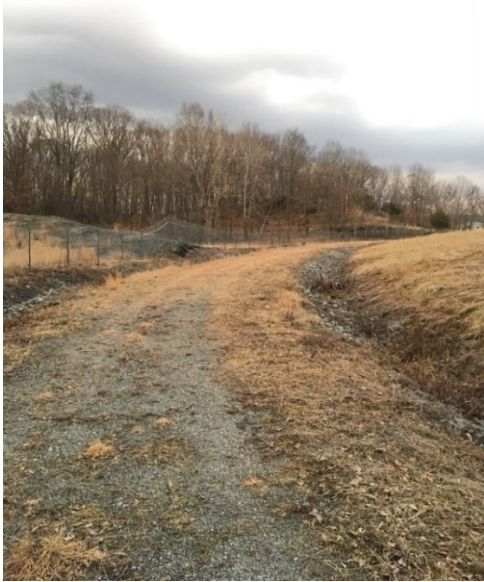
Photo 5: Looking east from the west side of the landfill. View of drainage swales on the western side of the site.
