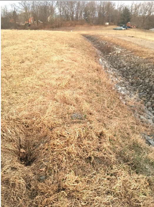
Photo 11: Looking east towards monitoring wells S-1 and B-1. View of drainage swale and landfill cap with animal burrow.
