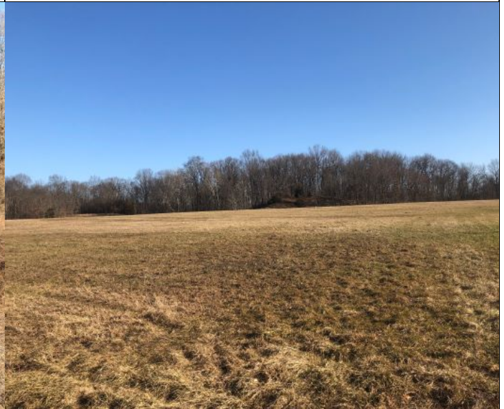
Photo 4: Overview of the landfill cap as taken from the southwest site boundary looking northeast.
