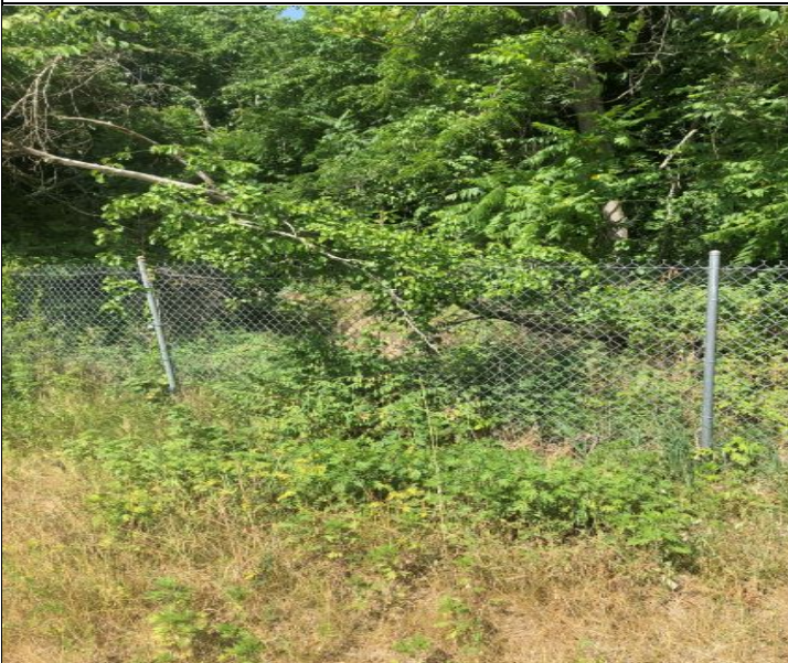
Photo 3: Tree that has fallen on the perimeter fence on the southern portion of the landfill.
