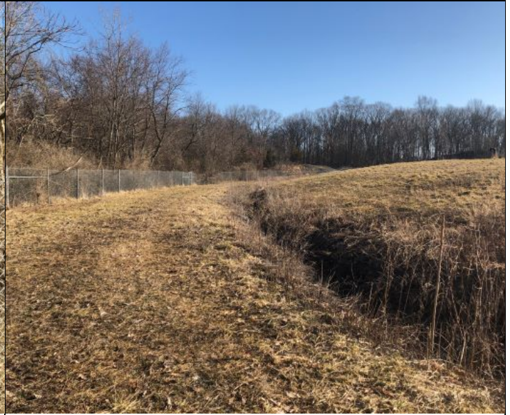
Photo 6: View of the northern fenced in Site boundary and drainage trench.
