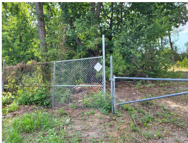
Photo 3 – View of the new fence section added in by PES, with the tree cut down and cleared.
