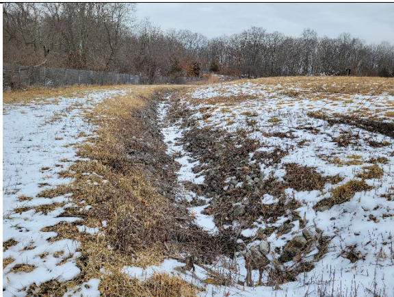
Photo 5 – Looking east at swale located in northern portion of landfill.
