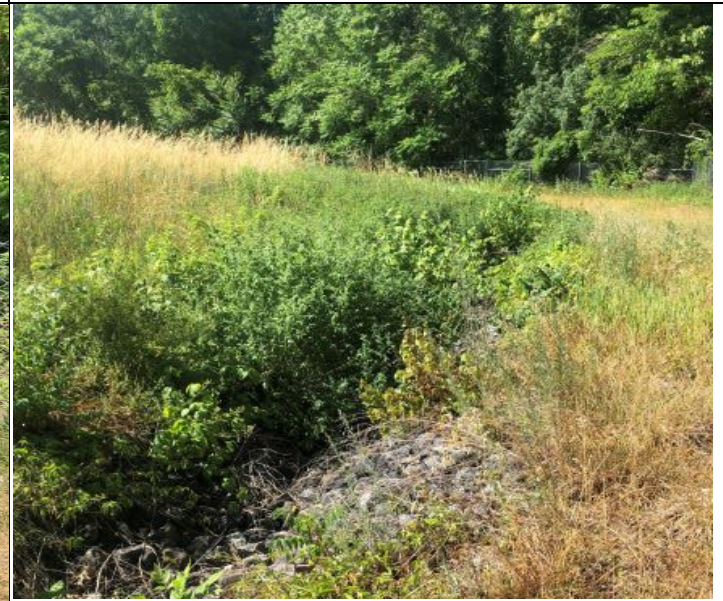
Photo 4: Thick vegetation located in the drainage areas near the southern portion of the landfill
