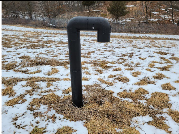
Photo 7 – Looking north typical landfill gas vent observed during inspection.
