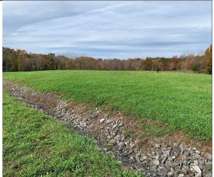
Photo 4: Overview of the landfill cap as taken from the north-east site boundary looking south-west.
