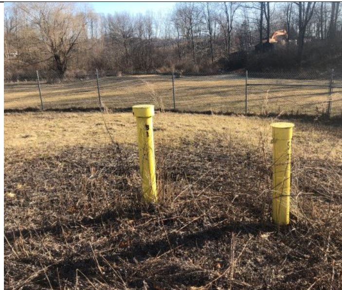
Photo 7: Monitoring wells B-1 and S-31 located at the northeast corner of the site. View looking northeast.
