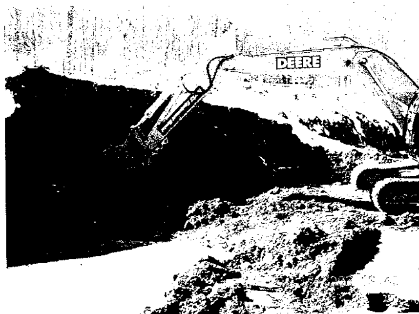
DSCN0143: Excavation along the west side of the excavation area looking north.
