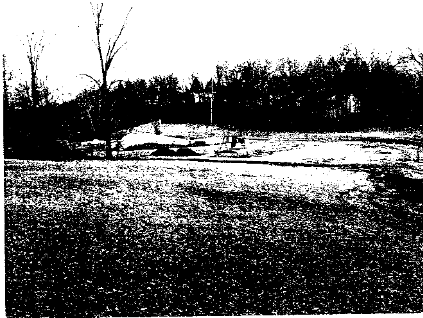
DSCN0197: Looking northeast toward the Trash Pile "D" area during backfilling
