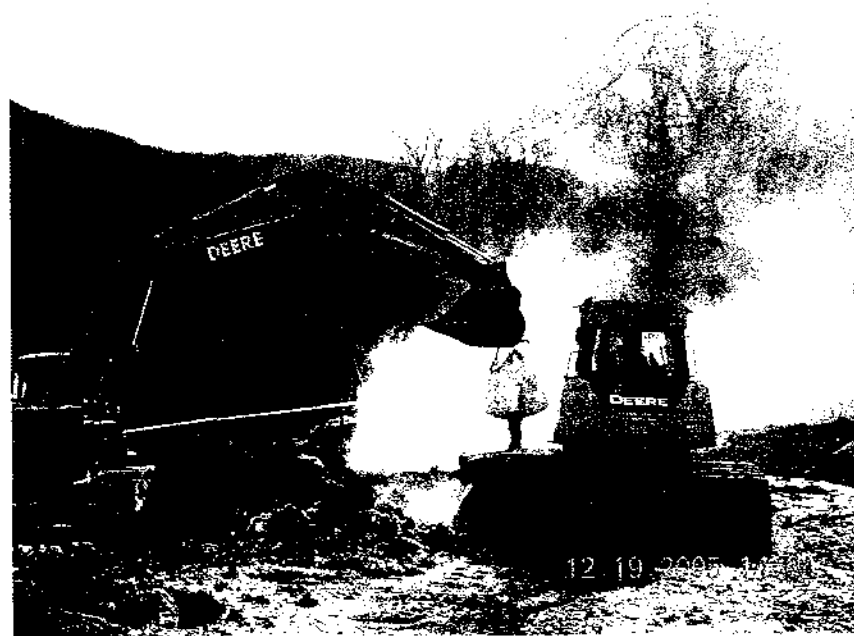
DSCN0065: Mixing the powdered bentonite with the soil prior to placement as a cutoff wall.
