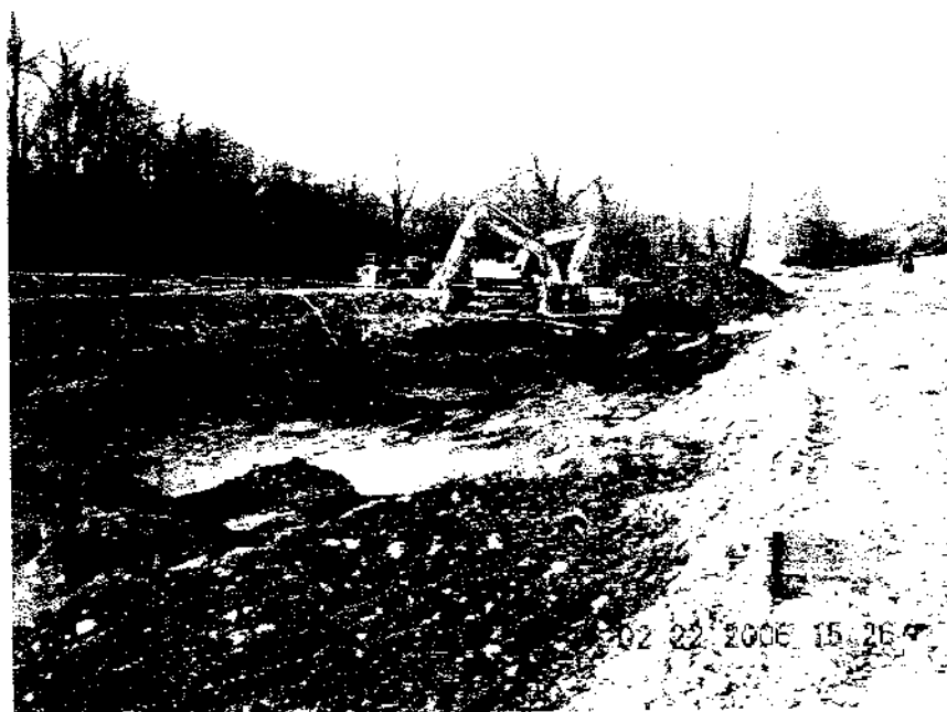
DSCN0168: Looking north toward continuing excavation.
