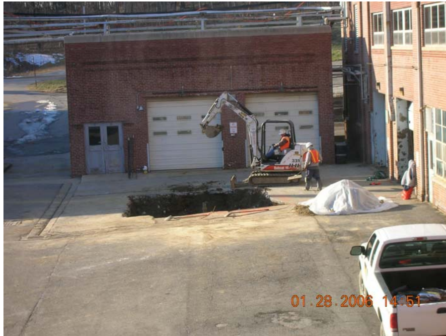
DSCN0117: Excavation of Building 56 cleanout
