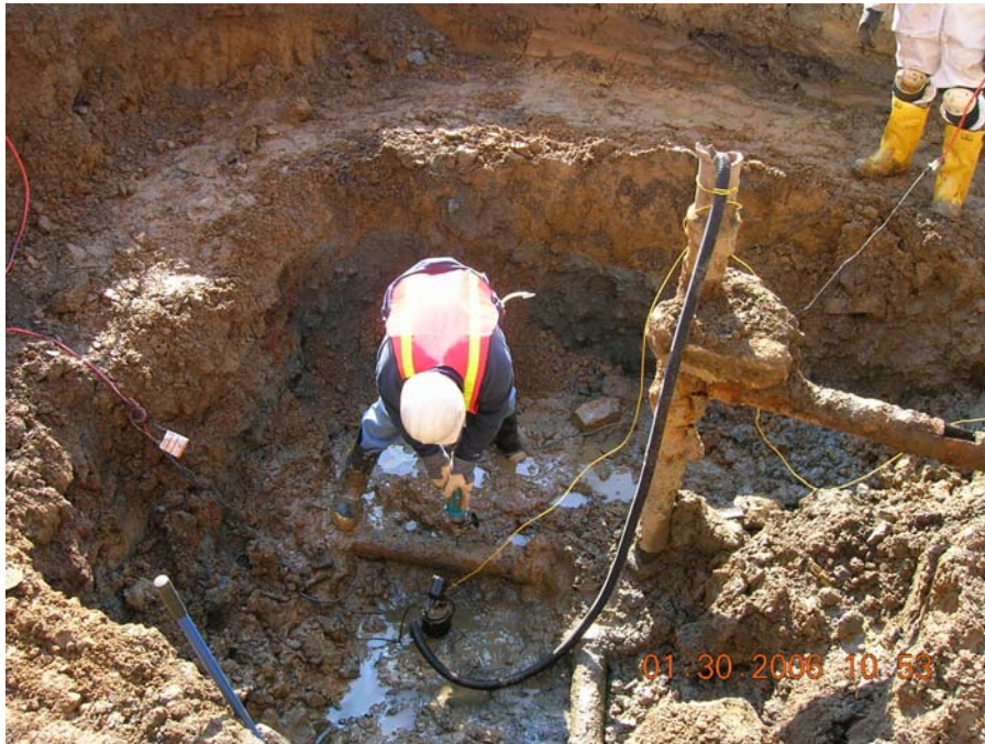
DSCN0122: Building 56 cleanout assembly
