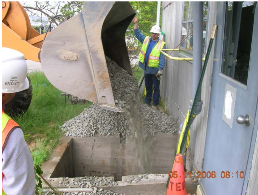
DSCN0359: Backfilling Building 42 vault (A-line).
