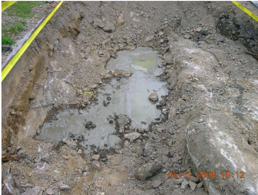
DSCN0378: ISS-5 excavation grouted.
