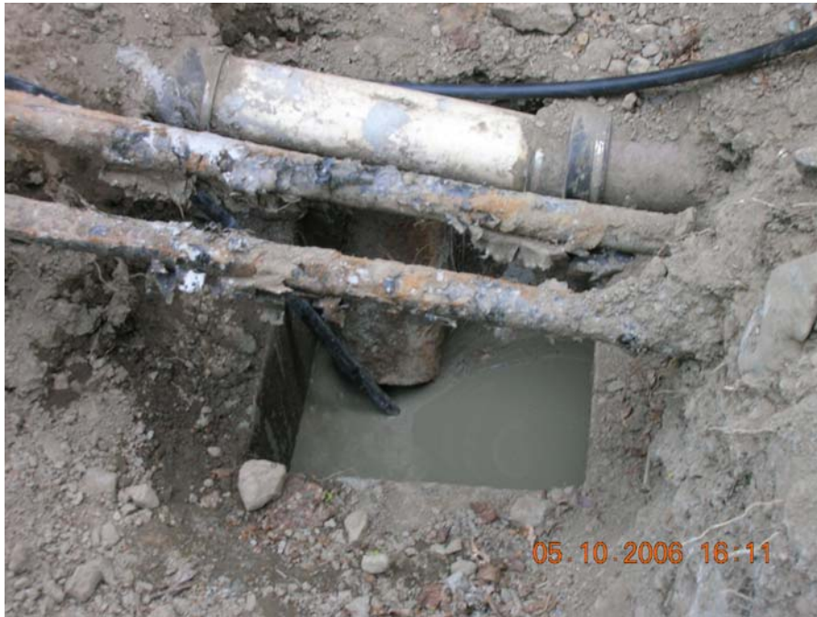
DSNC353: Grouting the 3x3 vault south of Building 55. (ISS-5, B-line)
