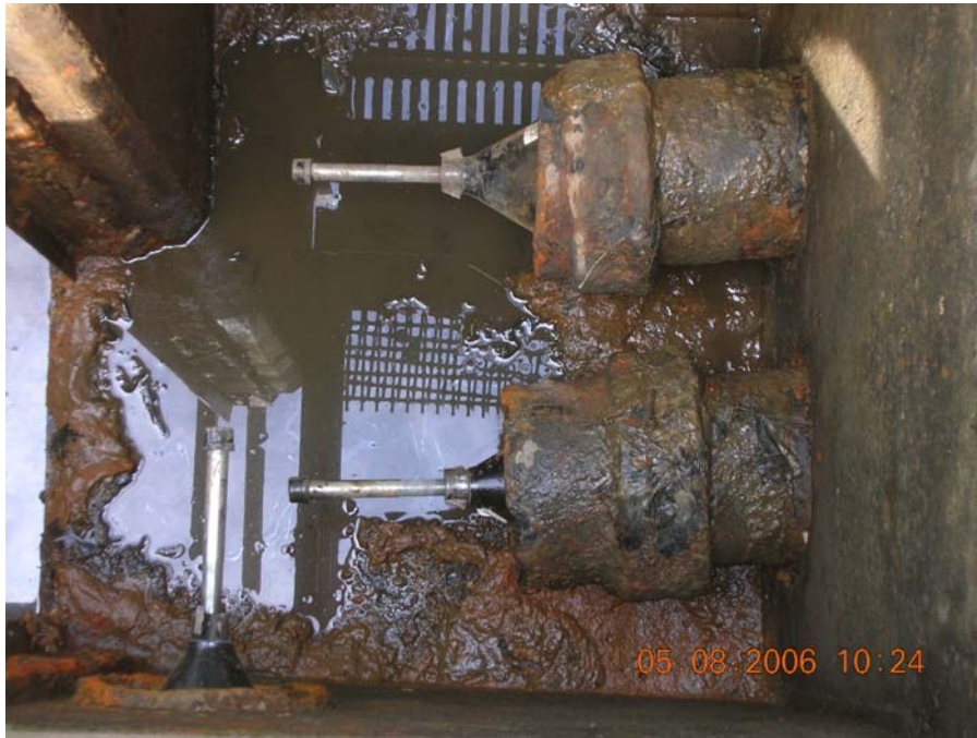
DSCN0303: Plugged outlets to the grit chamber. ISS-5, ISS-6, ISS-8.
