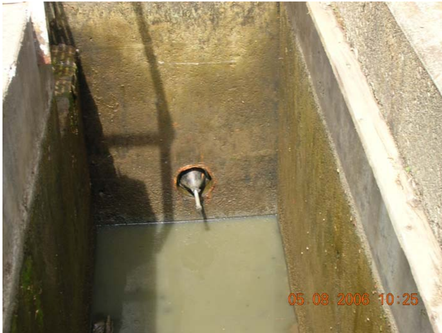
DSCN0304: Plugged outlet to the grit chamber. A-line.
