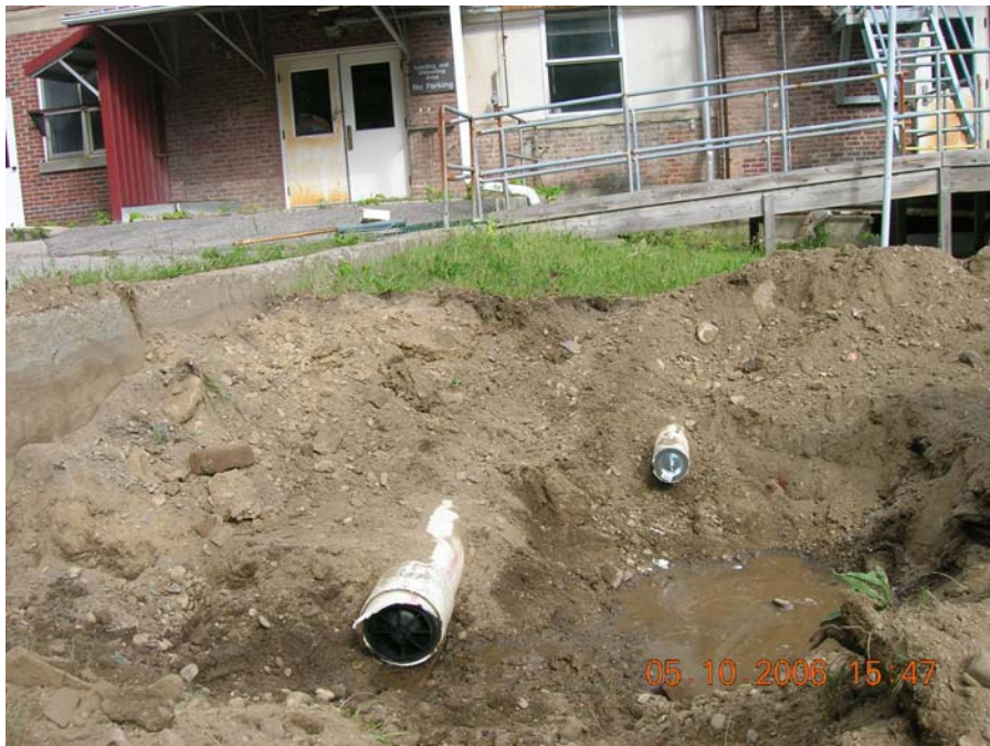
DSCN0349: Plugged PVC lines from ISS-7.
