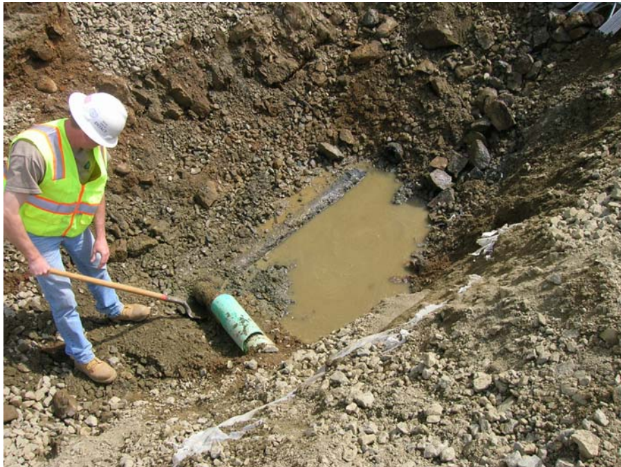
DSCN0281: Failed connection from Building 56 wash rack area.
