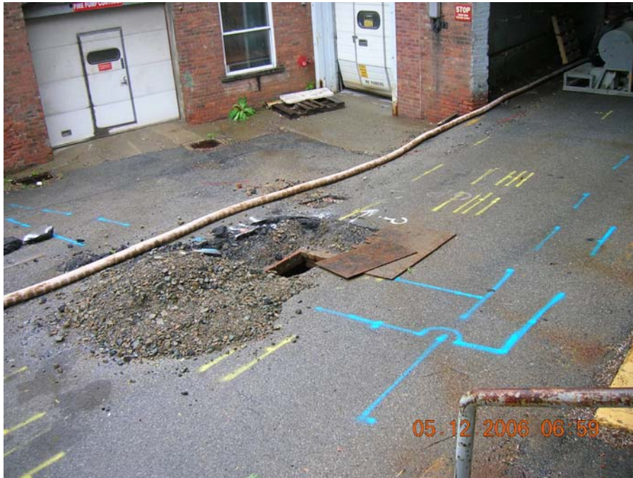
DSCN0380: 3x3 sewer pit on ISS-8 line.
