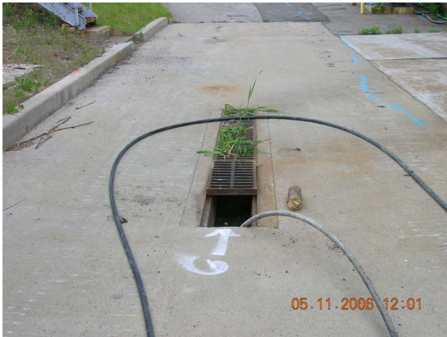
DSCN0366: Grouting spill containment basin for boiler house ASTs. (ISS-5)
