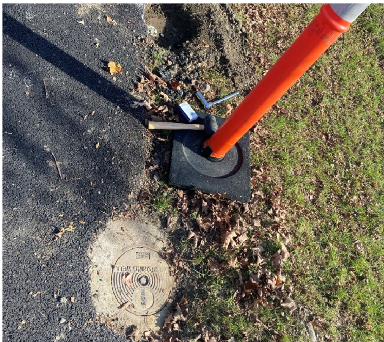
4. OS-3/OR-3. Recent paving buried OR-3. Located with metal detector and exposed.
