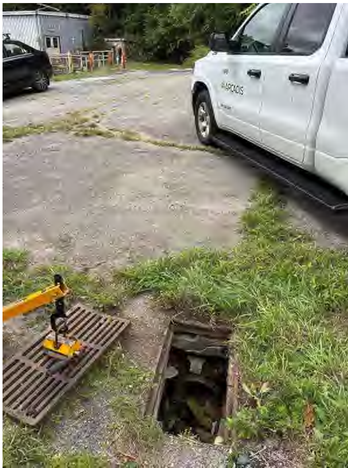
Photo Caption | Storm drain near 45. 8" ceramic outlet towards NW. 2" pvc inlet
