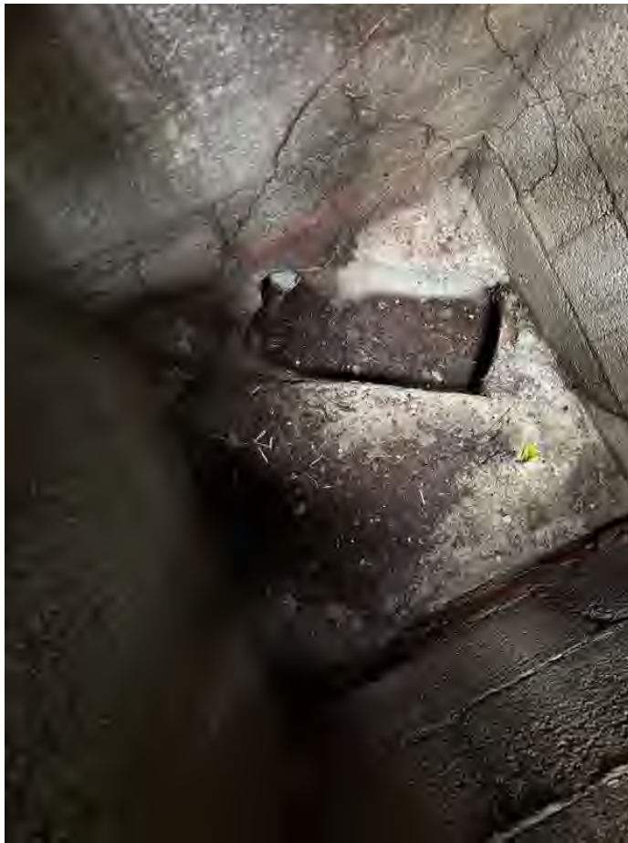
Photo Caption | Inlet 10" ceramic from NE. Outlet 10" ceramic 45 degrees into building towards S
