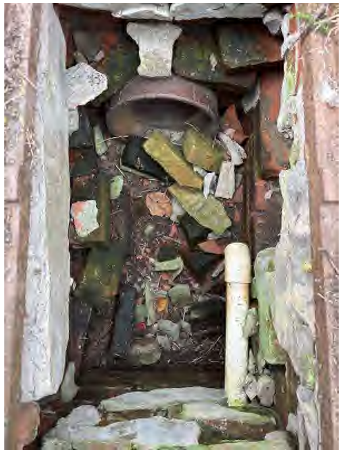
Photo Caption | Storm drain near 45. 8" ceramic outlet towards NW. 2" pvc inlet
