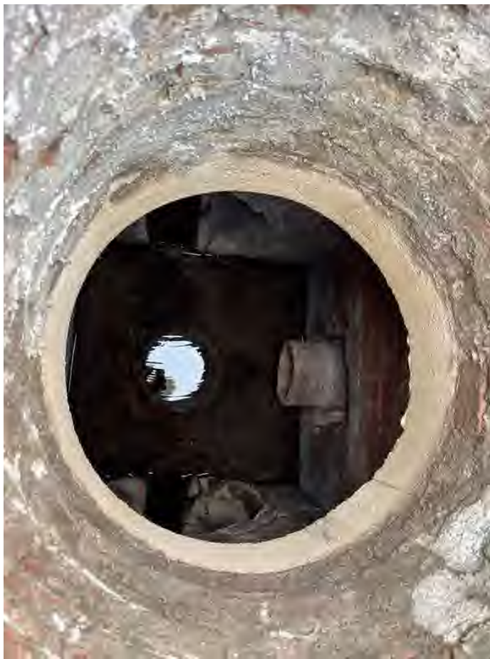
Photo Caption | Storm water manhole 90' from creek. 24" inlet & outlet. 8" inlet from SE
