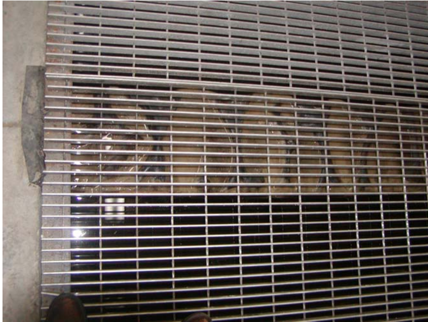
Weir between Sediment Tanks 1 and 2
