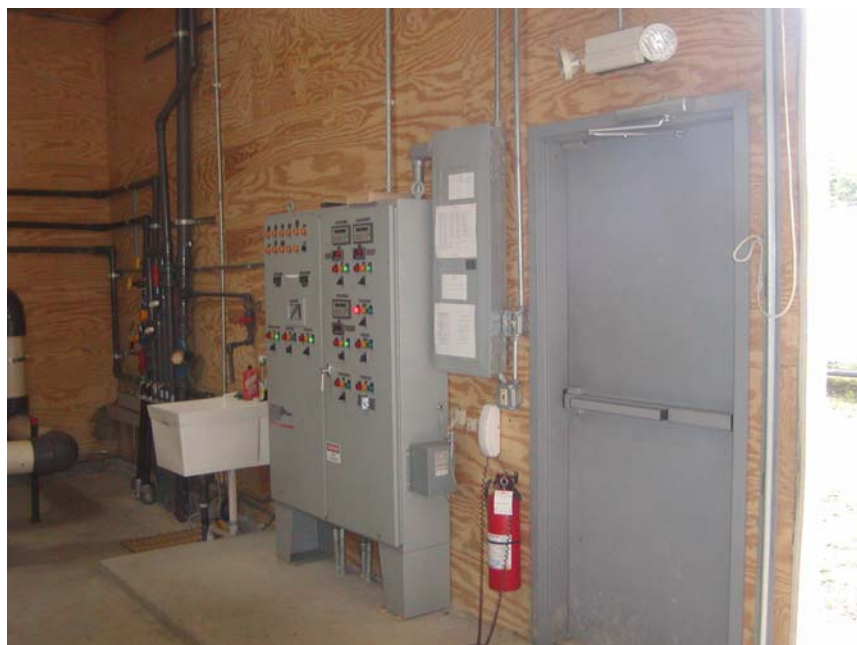
Treatment building view
