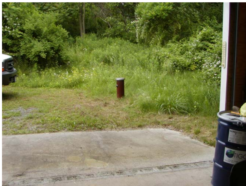
TW-2 extraction well outside building
