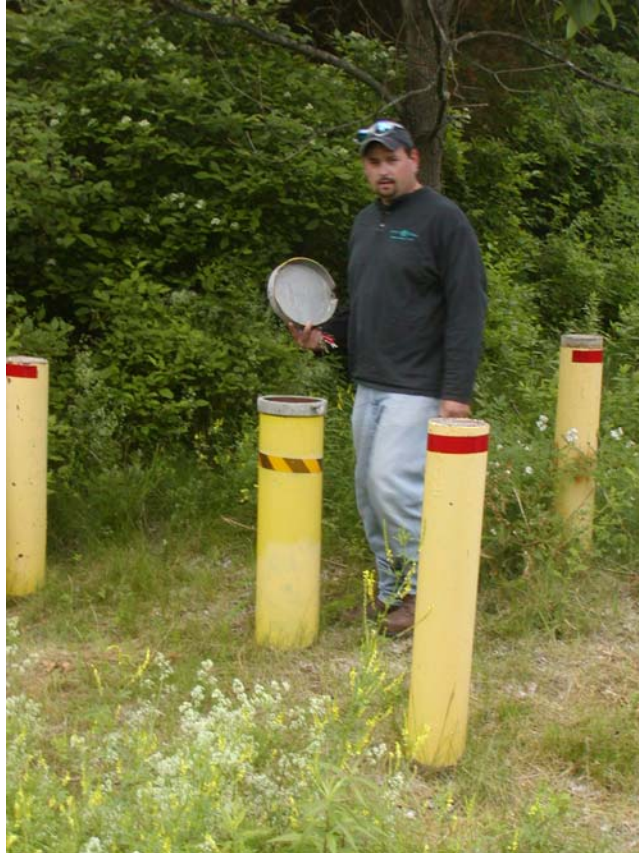
Infiltration well IW-1 (near effluent meter pit)
