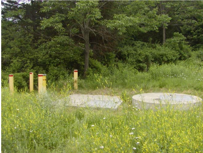
Distribution and meter pits and infiltration well, looking NE
