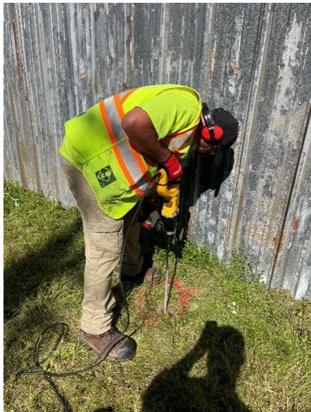
AECOM employee hammer drilling to prepare ground for soil vapor passive sampling point.
