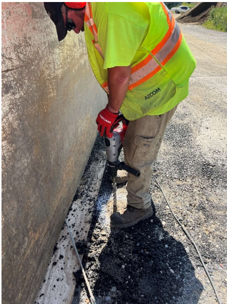
AECOM employee drilling hole for soil vapor sample media installation.
