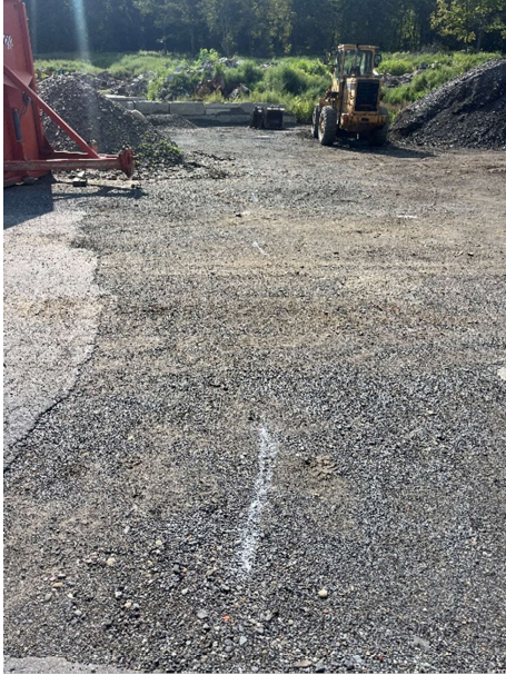
AECOM marked out the boundary of the GPR survey using a white dashed line.
