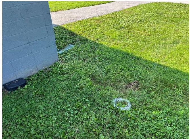
AECOM began marking out proposed soil vapor points with spray paint.
