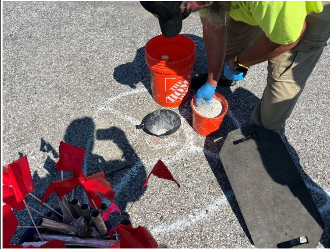
AECOM employee backfilling soil gas sample locations with bentonite chips.
