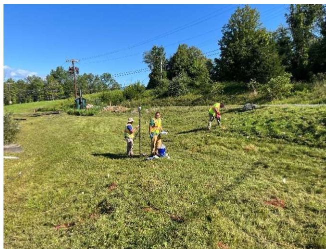
AECOM employees installing soil vapor sampling media.
