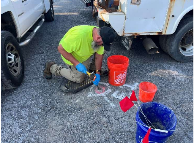
AECOM employee using bull point to chip through concrete seal at soil gas sample location.
