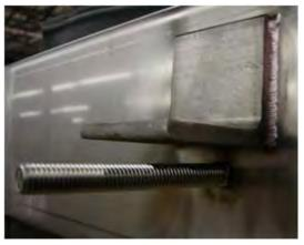
**2.** Remove the knobs and latches from the bolts above and below the door.
