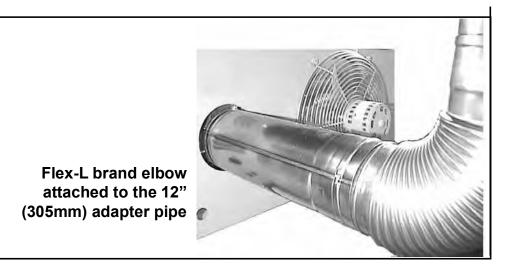
If using a 4" (102mm) diameter, 12" (305mm) long adapter pipe - Following the vent pipe manufacturer's instructions, attach one of the following:
