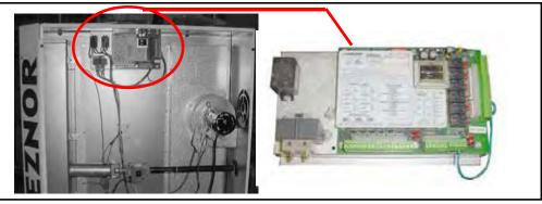
Control **Option D10** includes the controller and the sensor to be field mounted at the heater discharge. **Option D14** requires a field-supplied sensor that is compatible with the control. For regulatory compliance specifications, and safety precautions, review the control manufacturer's installation instructions in the owner's envelope.
