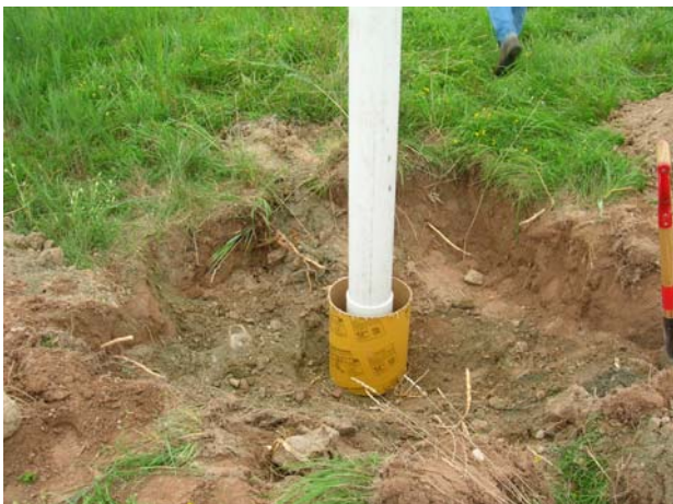
The existing pipe is cut and a new Riser is added. Then a Sauna Tube is put around the base.
