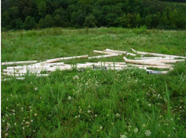
Existing PVC collection system which was lying on top of the ground was cut up and stacked
