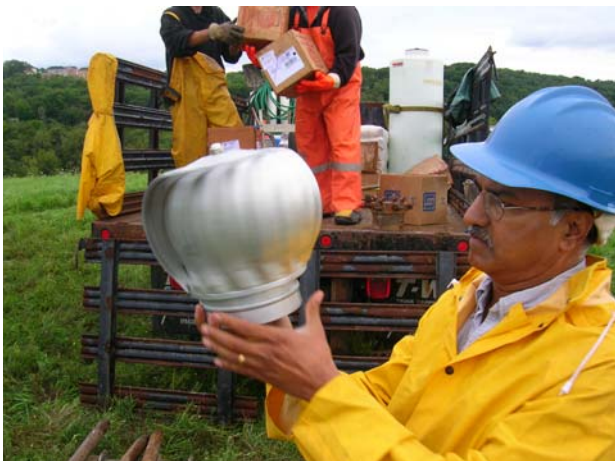
One of the Turbine Ventilators
