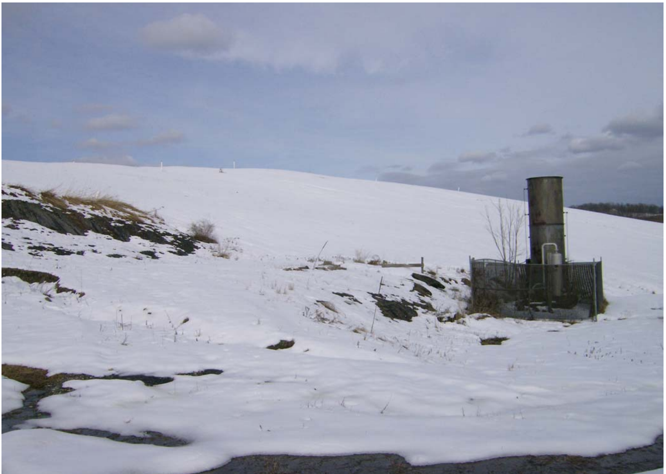
March 2010 photo of FICA landfill. Turbine vents at summit of landfill and former used totally enclosed flare in foreground. No problems evident during DER staff site visit, however significant snow cover was present.
