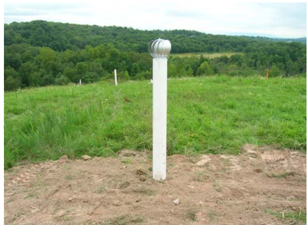
Finally the soil is backfilled and leveled around the Converted Vent
