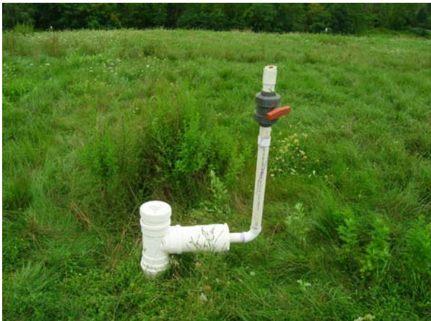
Sections of PVC pipe with the original valves were re-attached after disassembly of the system
