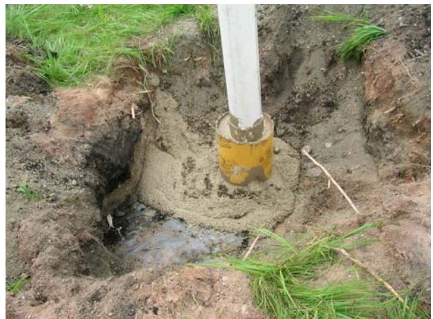
The Sauna Tube is filled with concrete
