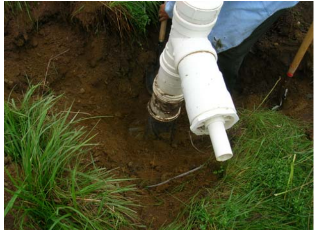
The hand shovel is used to expose the boot to prevent damage to the liner
