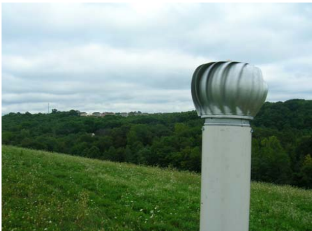
A close up of the Turbine Ventilator at the top of the Riser
