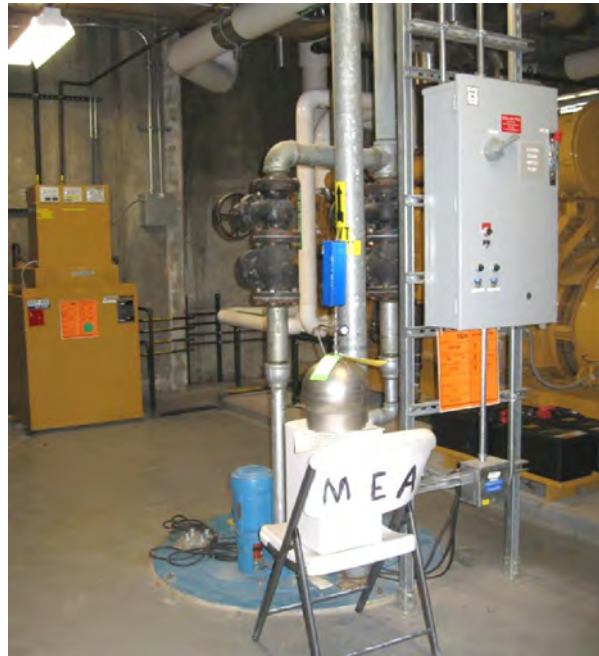
PHOTO #2 – Sample IA-0801; located near a stormwater sump for the subgrade HVAC intake in room with backup generators.
