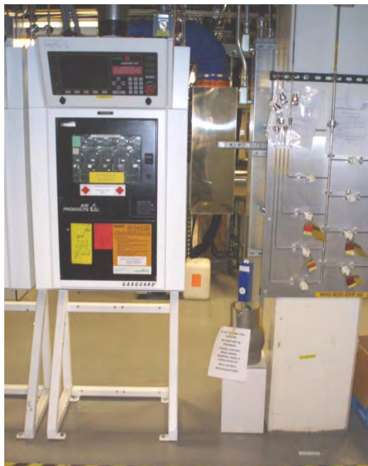
PHOTO #5 – Sample IA-0804; located in the sub-fab area.
