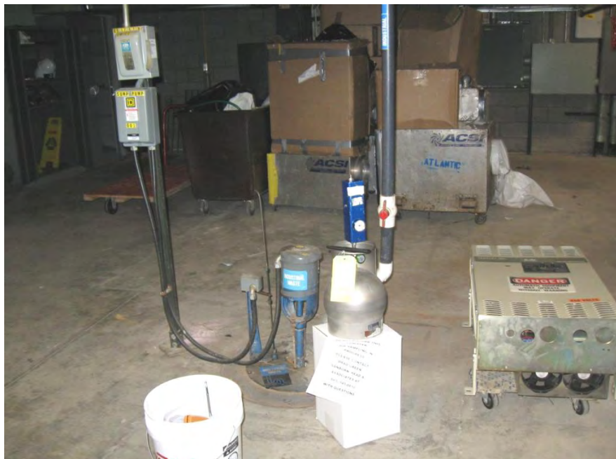
PHOTO #9 – Sample IA-1008; located near a sump in a mechanical room.
