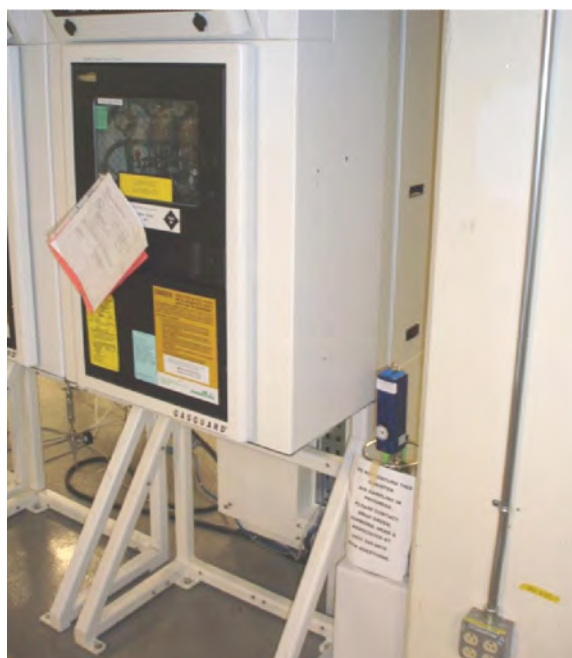
PHOTO #8 – Sample IA-0807; located in the sub-fab area.
