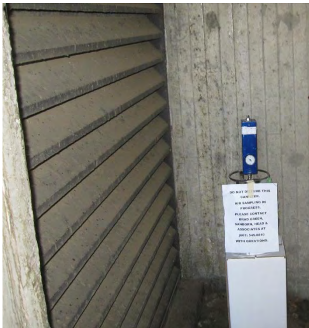
PHOTO #11 – Sample AA-1010; located near the AC-D6 HVAC intake on the north side of the building.
