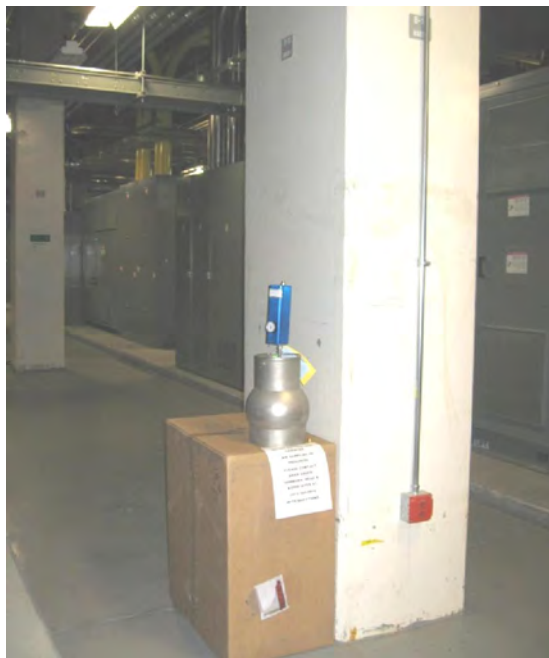
PHOTO #1 – Sample IA-0800; located in east electrical room.
