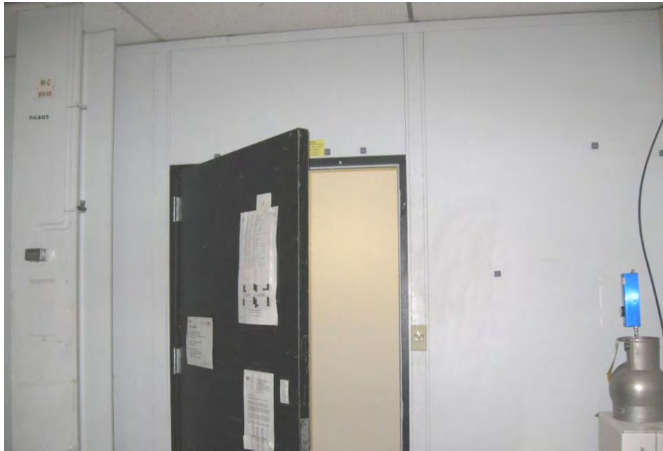
PHOTO #2 – Sample IA-1001; located in an unoccupied office.
