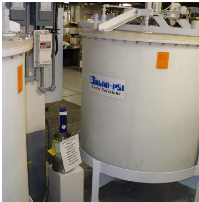
PHOTO #6 – Sample IA-0805; located in the sub-fab area near an above ground storage tank (AST) containing copper.
