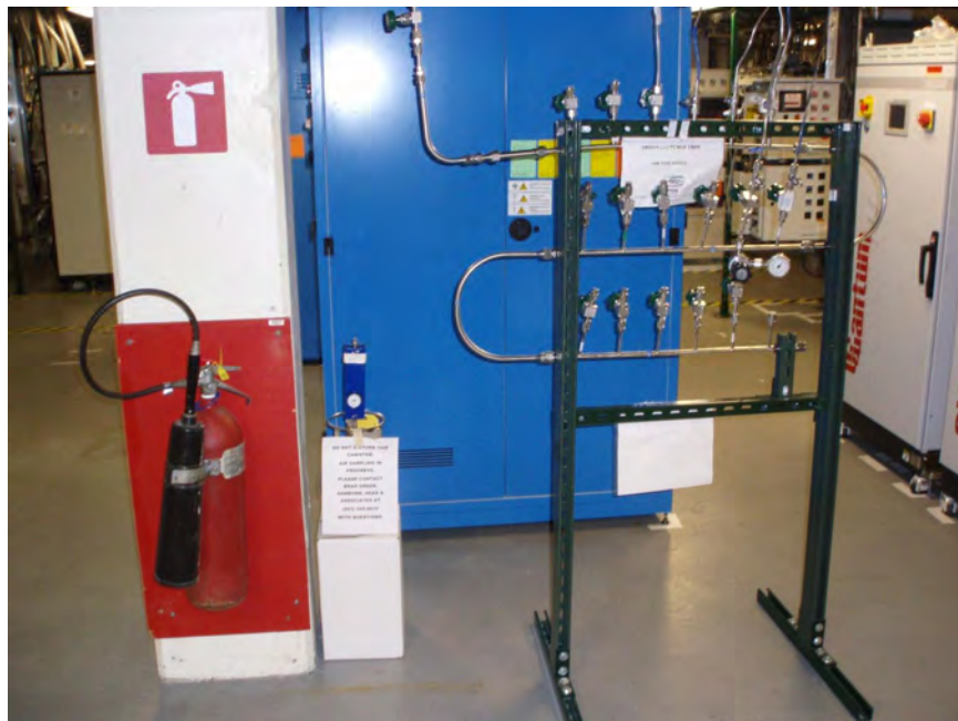
PHOTO #7 – Sample IA-0806; located in the sub-fab area next to exhaust units.
