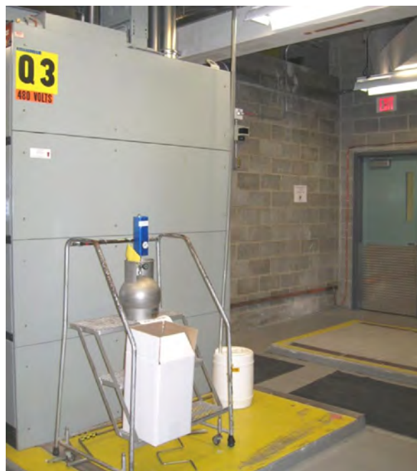
PHOTO #16 – Sample IA-0815; located in the west electrical room.
