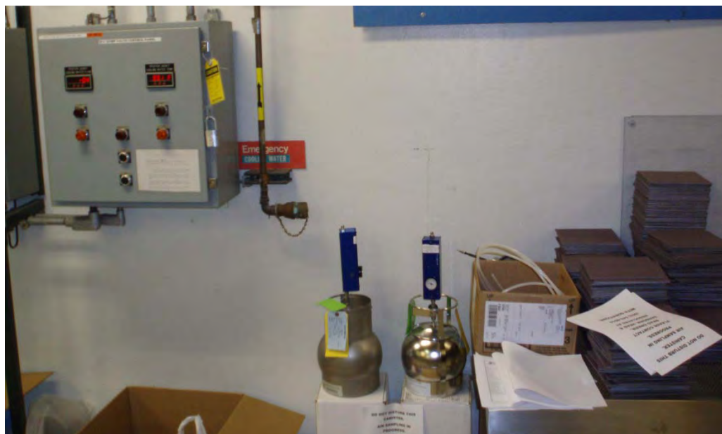
PHOTO #6 – Sample IA-0416 and Duplicate; located in the sintering manufacturing furnace room #2.
