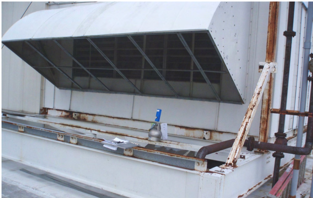
PHOTO #20 – Sample AA-0419; located near and intake to AC-13.
