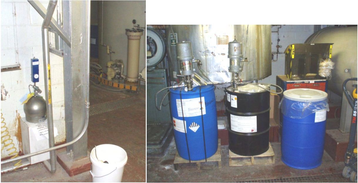
PHOTO #7 – Sample IA-0406 (left picture); located in a solvent management/drum storage area.
