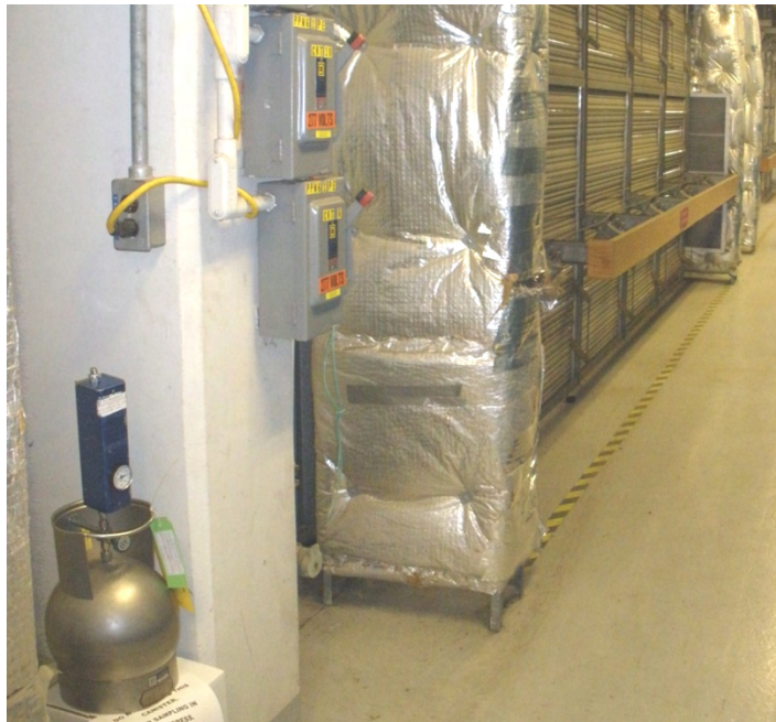
PHOTO #16 – Sample IA-0415; located on the southern side of the Sintering Manufacturing Furnace Room #2, near a wall of louvered doors.
