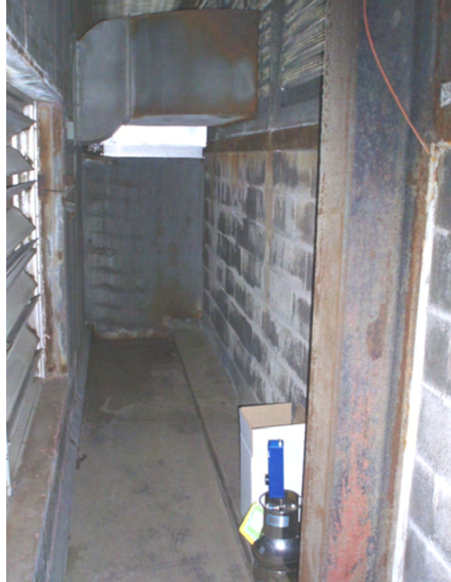
PHOTO #21 – Sample AA-0420; located in the plenum space near the AC-04 intake.
