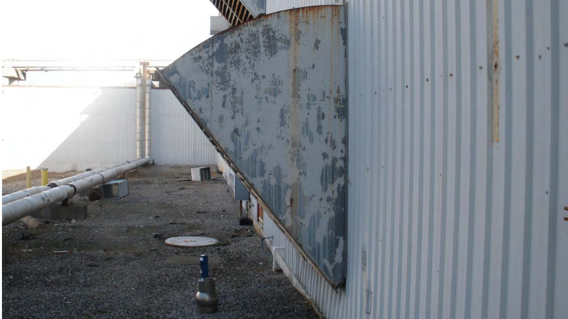
PHOTO #7 – Sample AA0106; located near the intake for AHU-11.
