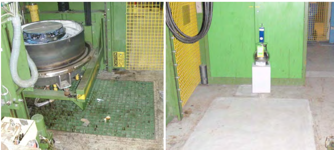
Exhibit H: Pit in the Sintering Room (Pre- and Post-Closure)
