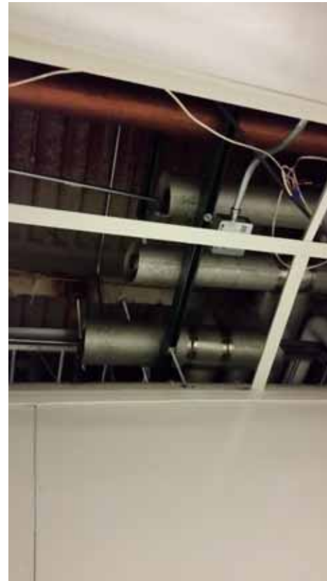
TMAH Pipe abandoned in place above ceiling between AY27-AZ29 in B 330D (approx. 60 ft.)
