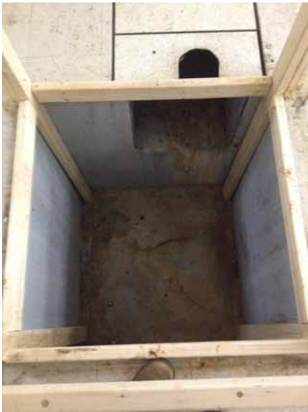
Cleaned Lift Station Pit
