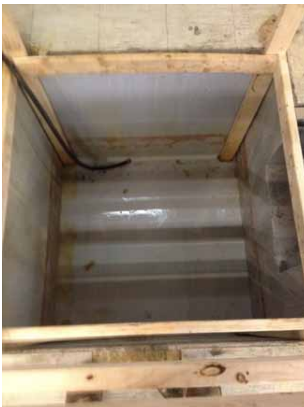
Cleaned Lift Station Pit
