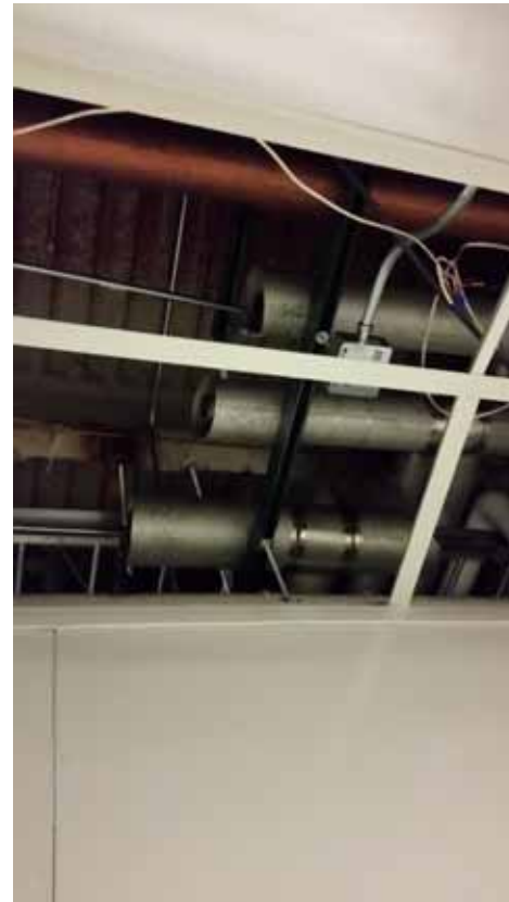
TMAH Pipe abandoned in place above ceiling between AY27-AZ29 in B 330D (approx. 60 ft.)
