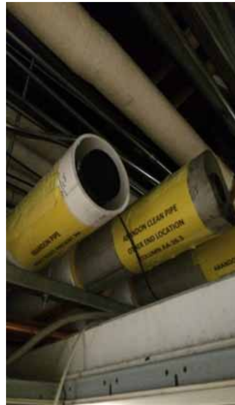
TMAH Pipe abandoned in place between AA26-AA31 in B 330C (approx. 120 ft.)
