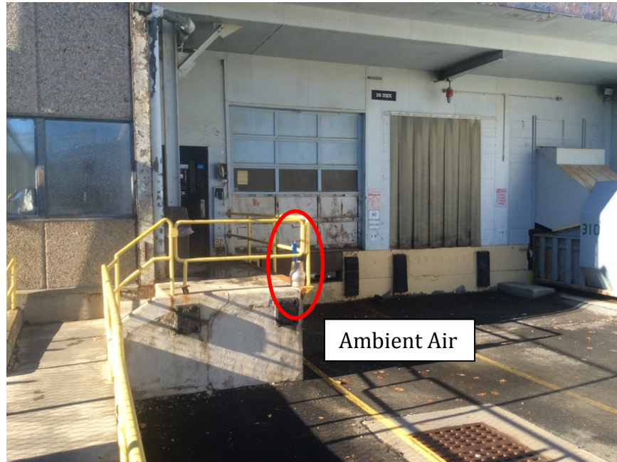
Photo 1: Ambient Air sample, B310 loading dock
