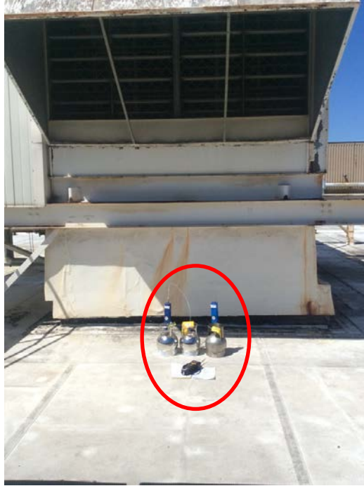
Photo 1: Samples AA0401 and FB0401 on roof of 330C at the intake for AC-58
