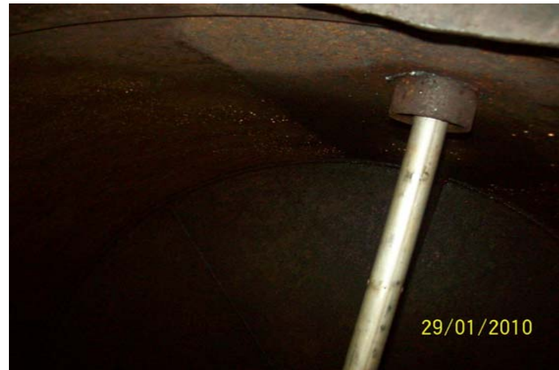
After Tank 207 was decontaminated.
