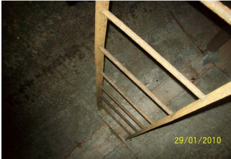
After Tank 204 was decontaminated.
