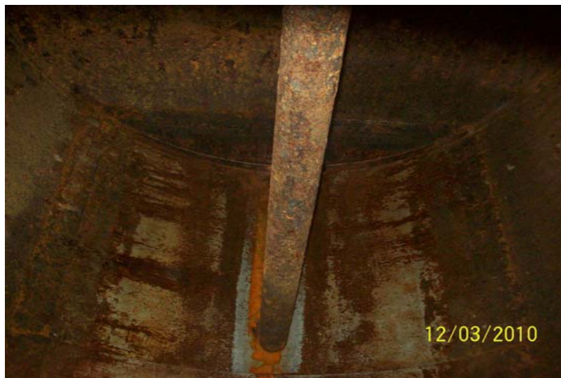
After Tank 205 was decontaminated a second time.
