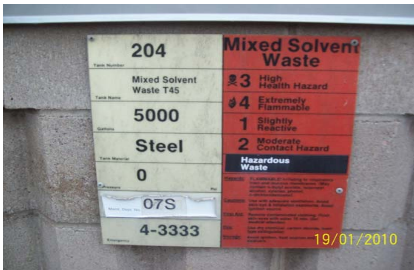
Tank 204 sign located on the exterior of the vault
