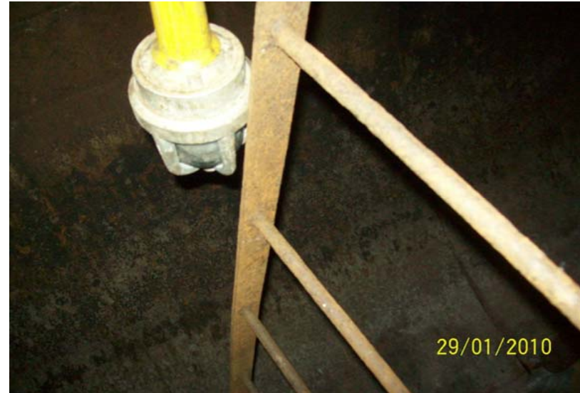
After Tank 204 was decontaminated.
