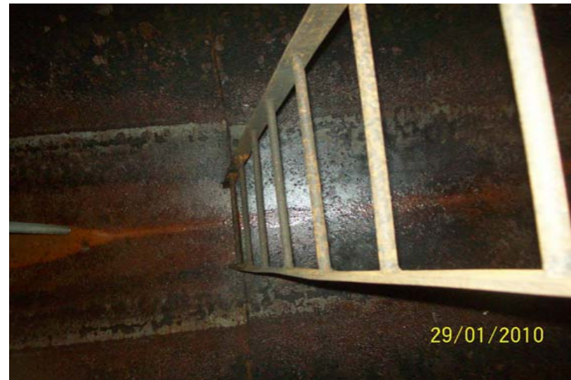
After Tank 206 was decontaminated.
