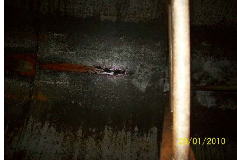
After Tank 207 was decontaminated.
