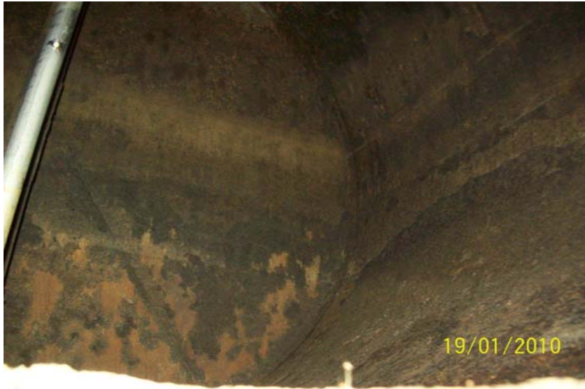
The interior of Tank 204
