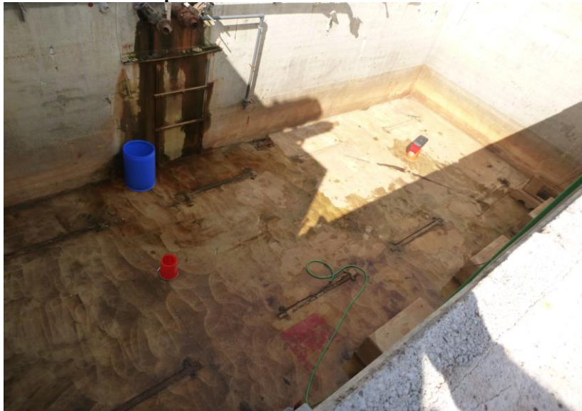
A view of the 2 rinse water sample locations within the Solvent Vault.
