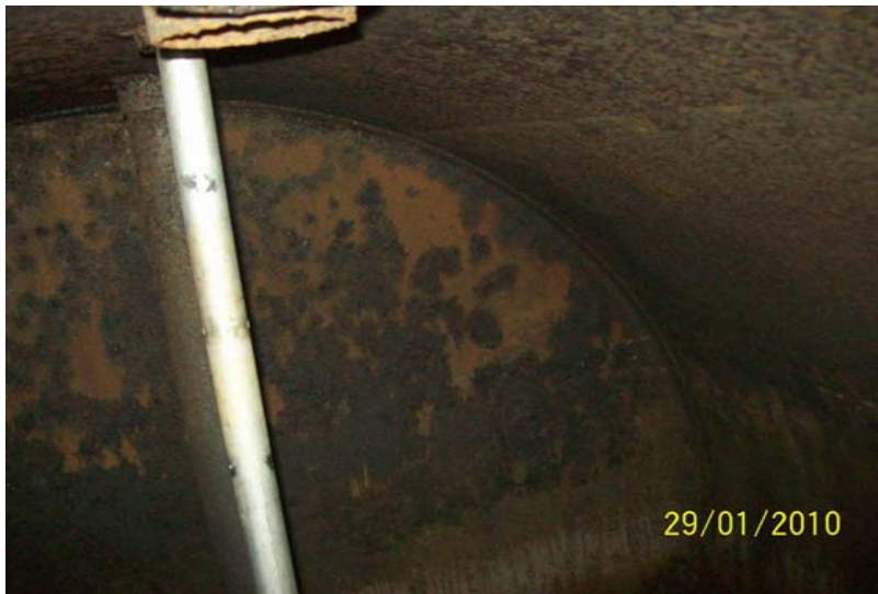
After Tank 204 was decontaminated.
