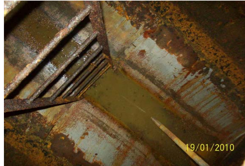
The interior of Tank 205
