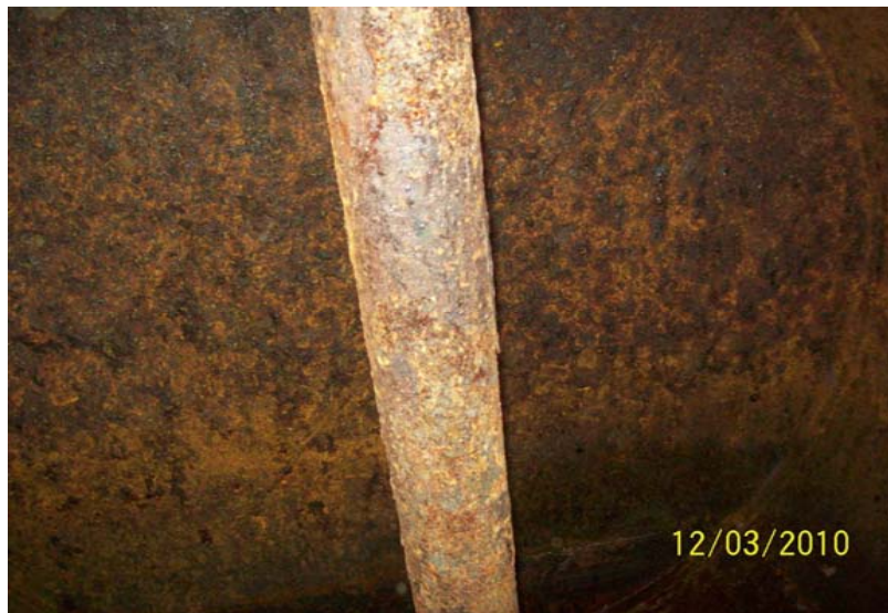
After Tank 205 was decontaminated a second time.
