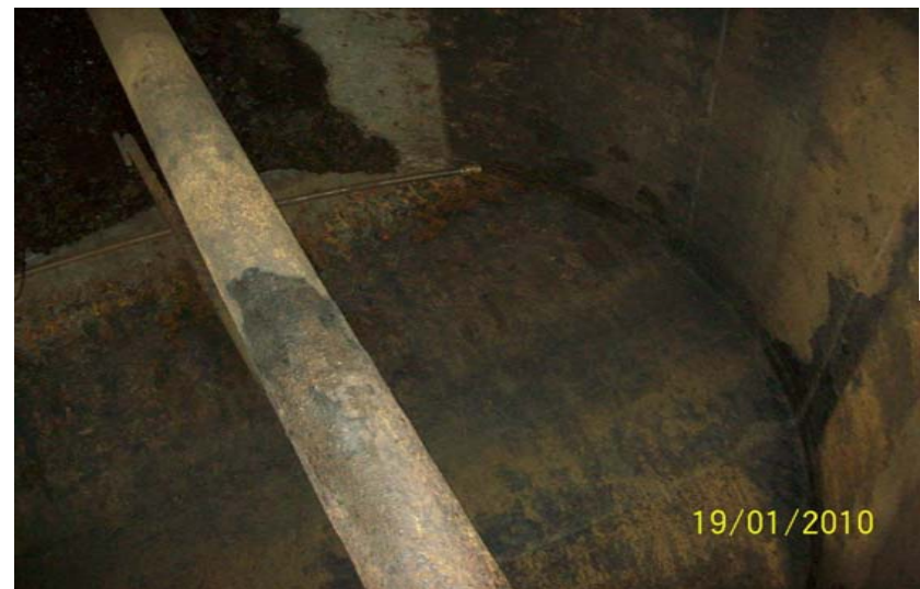
The interior of Tank 204
