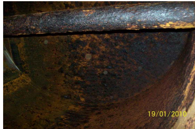
The interior of Tank 205
