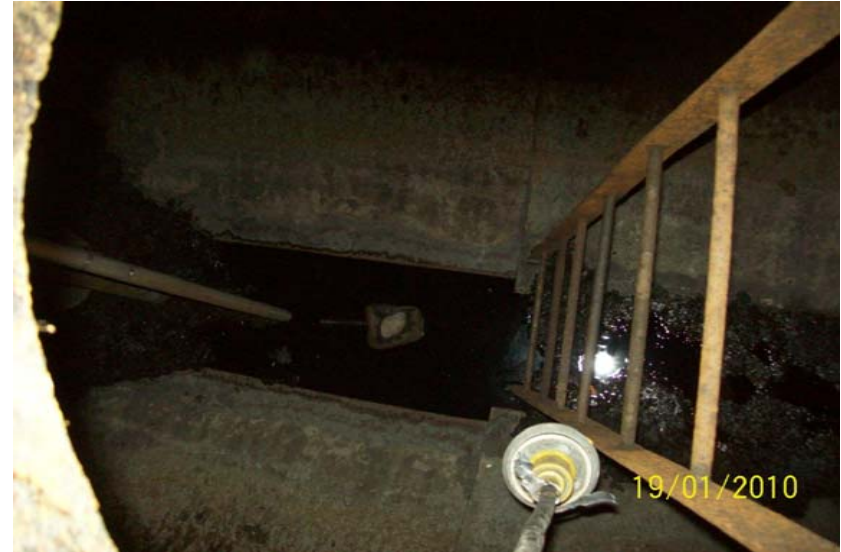
The interior of Tank 204
