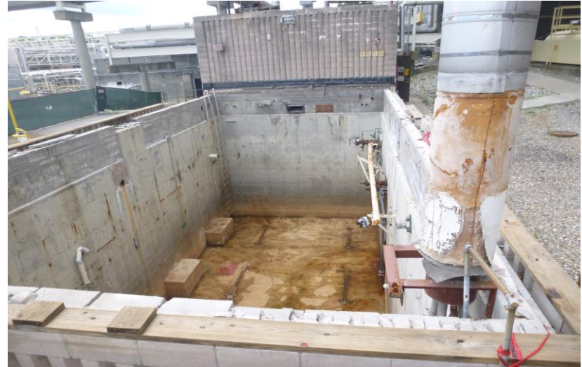
A view of the decontaminated Solvent Vault.
