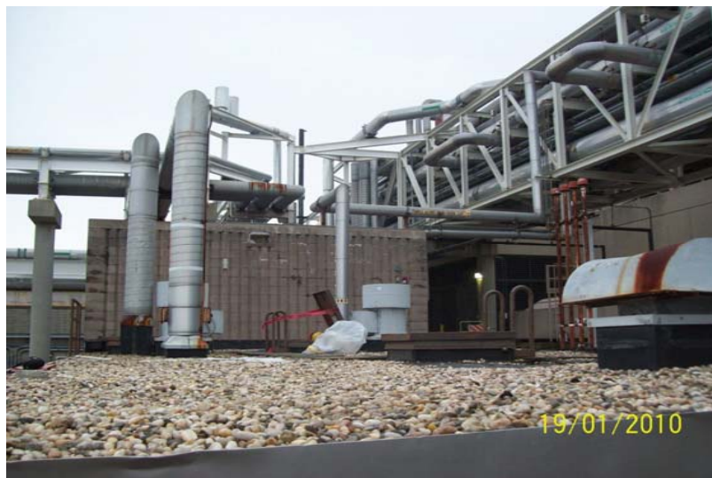
B/312B roof with access to the tanks through the roof hatches.
