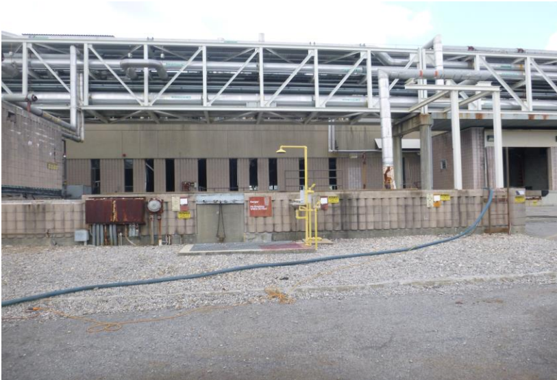
A view of B/312B Solvent Vault.
