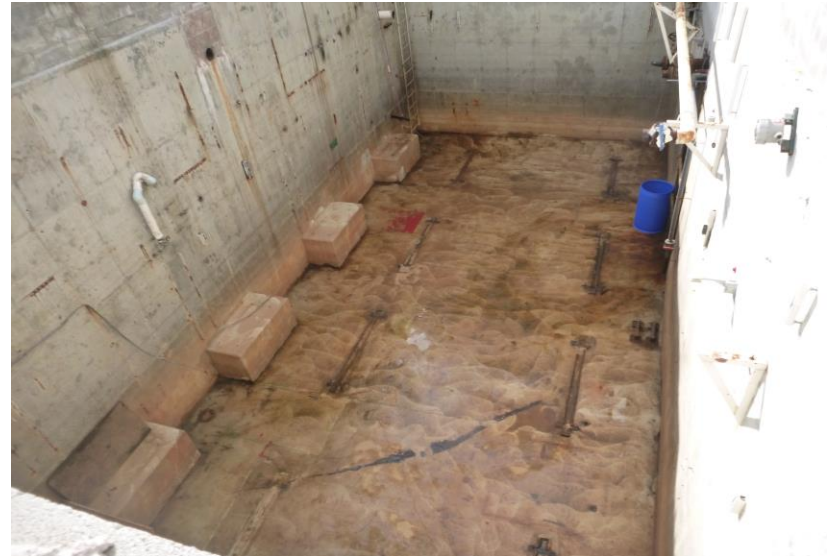
After the Solvent Vault was decontaminated.
