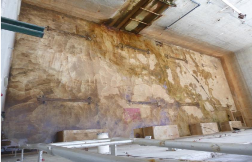
A view of the decontaminated Solvent Vault.
