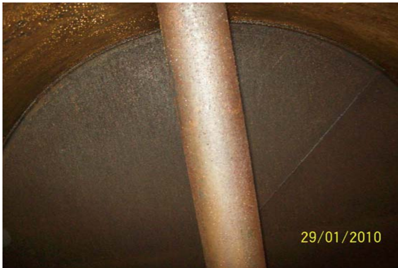
After Tank 207 was decontaminated.
