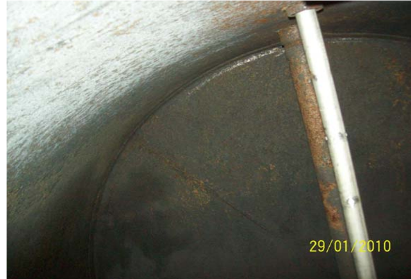
After Tank 206 was decontaminated.
