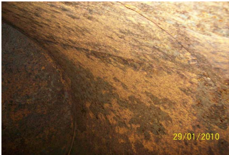
After Tank 205 was decontaminated.
