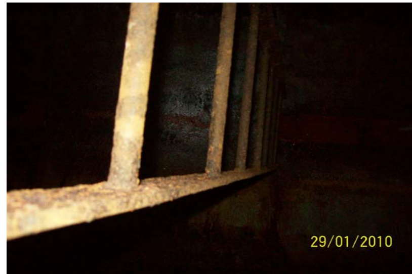
After Tank 205 was decontaminated.
