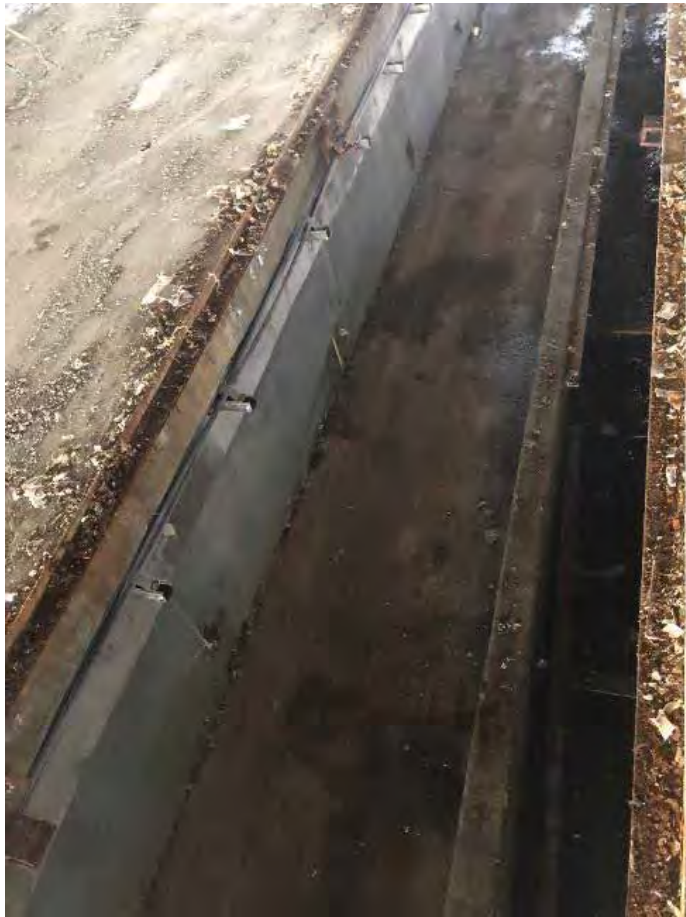
Cleaned Trench After Industrial Waste Pipe Was Removed
