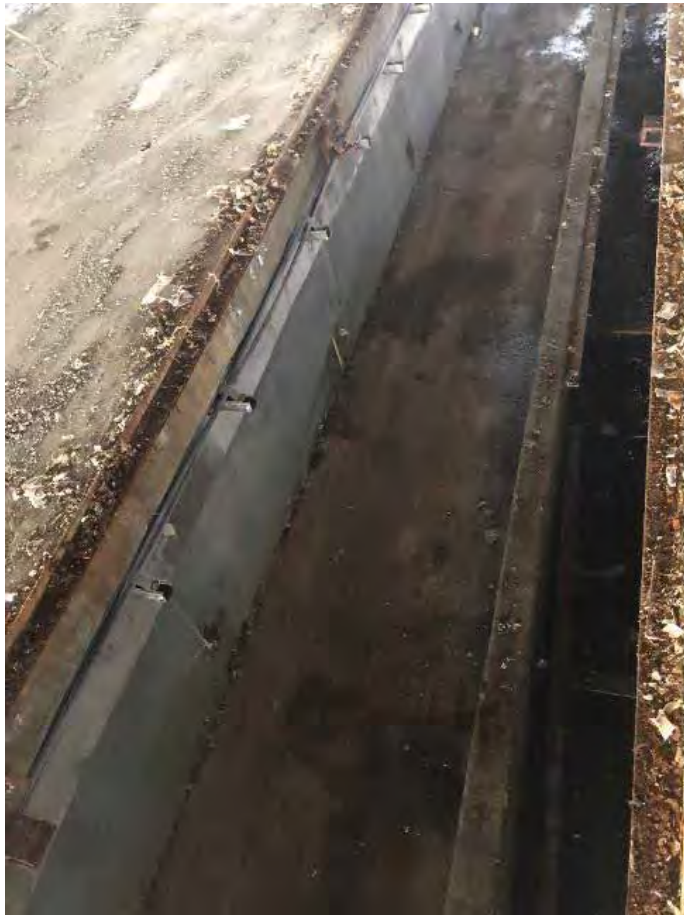
Cleaned Trench After Fluoride Pipe Was Removed
