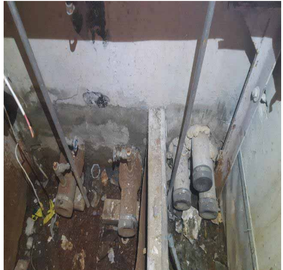
Fluoride Pipe Going Out Of Building Capped
