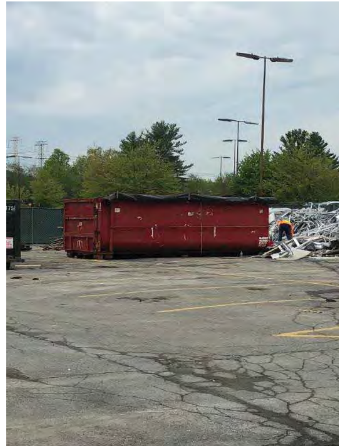
Roll-off Container For Hazardous Waste Solvent Pipe
