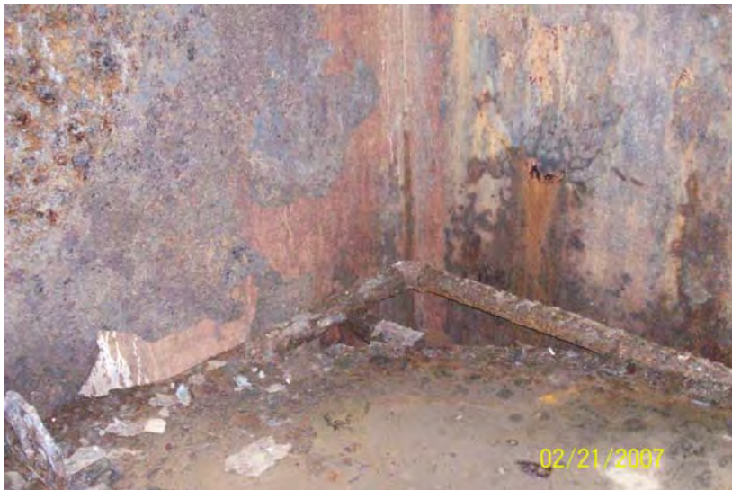
Rusted and corroded conditions within noted the stainless steel containment dike of Tank 208.
