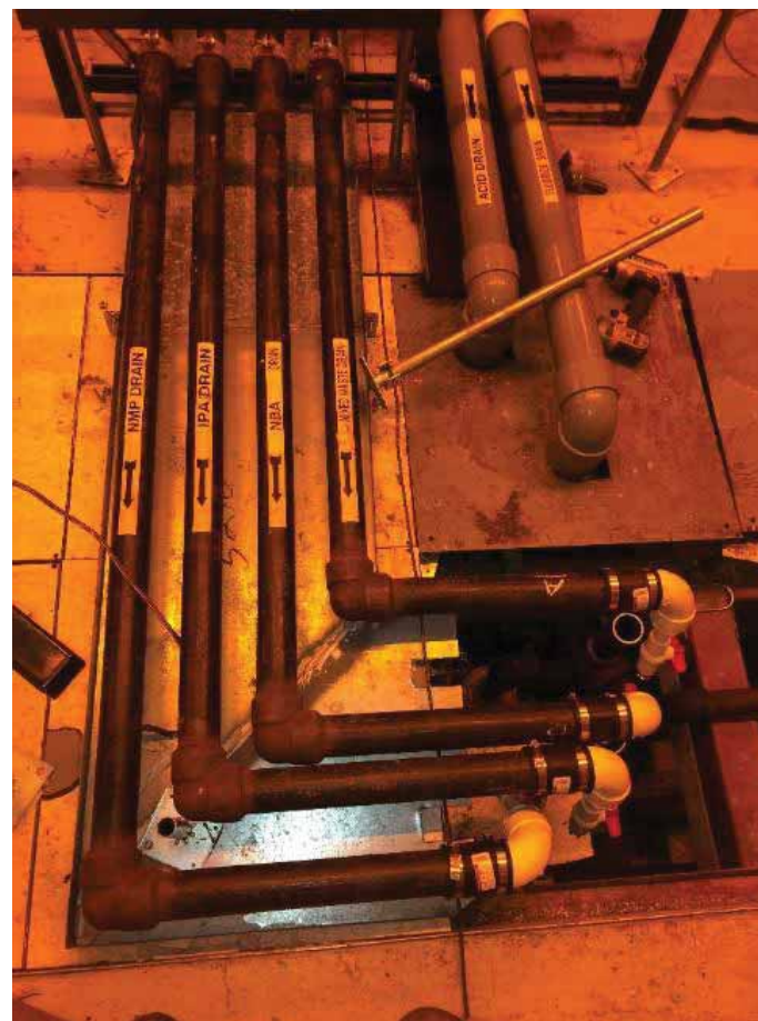
Solvent Pipe Pre-Removal
