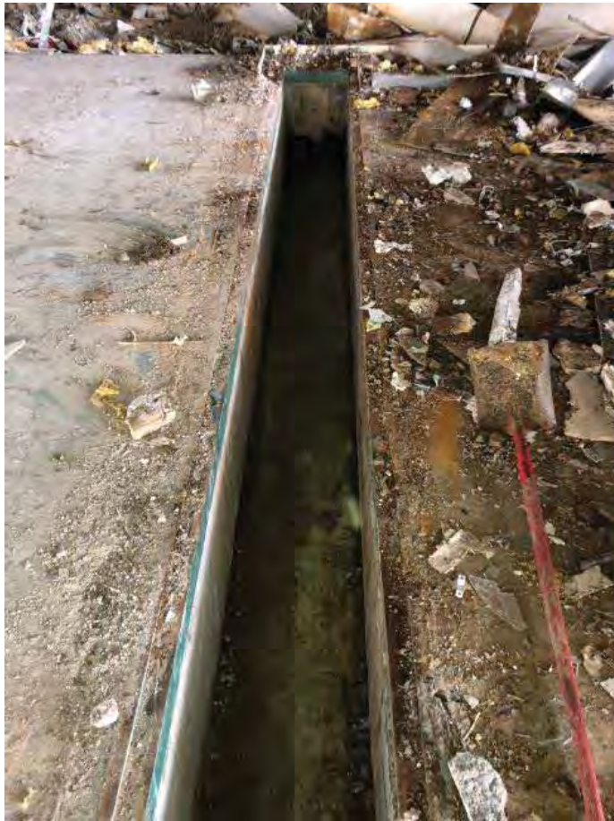
Cleaned Trench After Fluoride Pipe Was Removed
