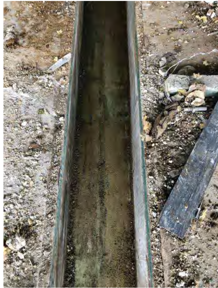
Cleaned Trench After Fluoride Pipe Was Removed
