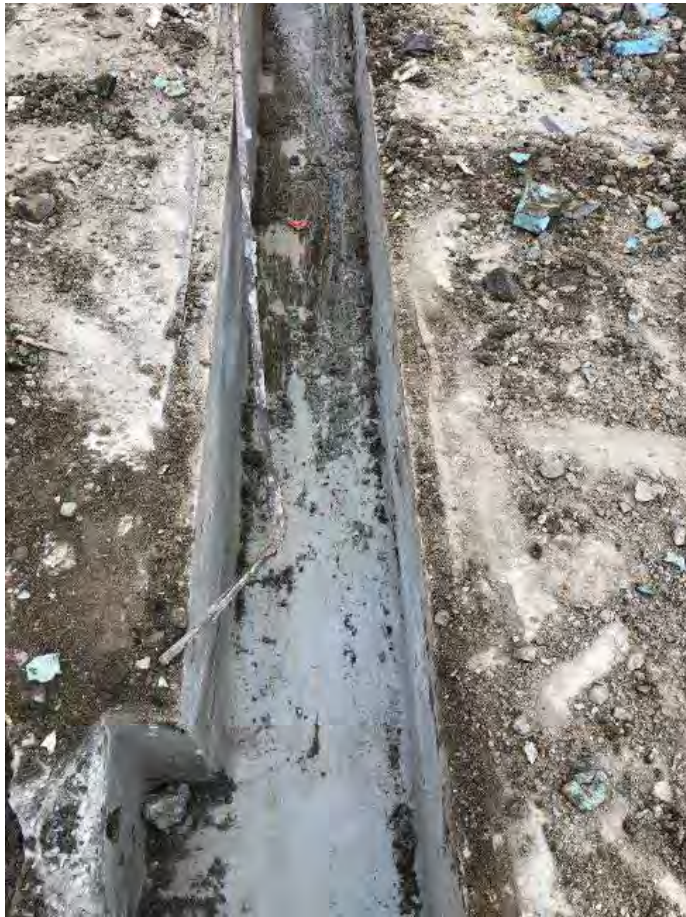
Cleaned Trench After Fluoride Pipe Was Removed
