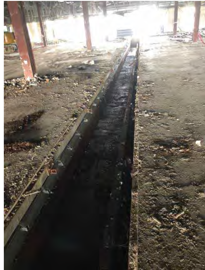
Cleaned Trench After Fluoride Pipe Was Removed
