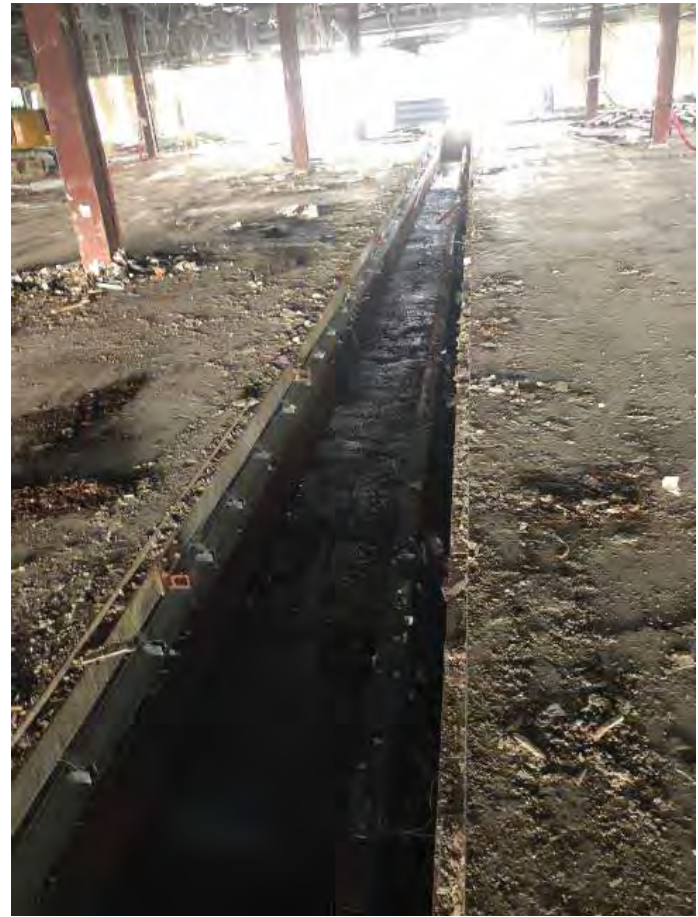
Cleaned Trench After Industrial Waste Pipe Was Removed
