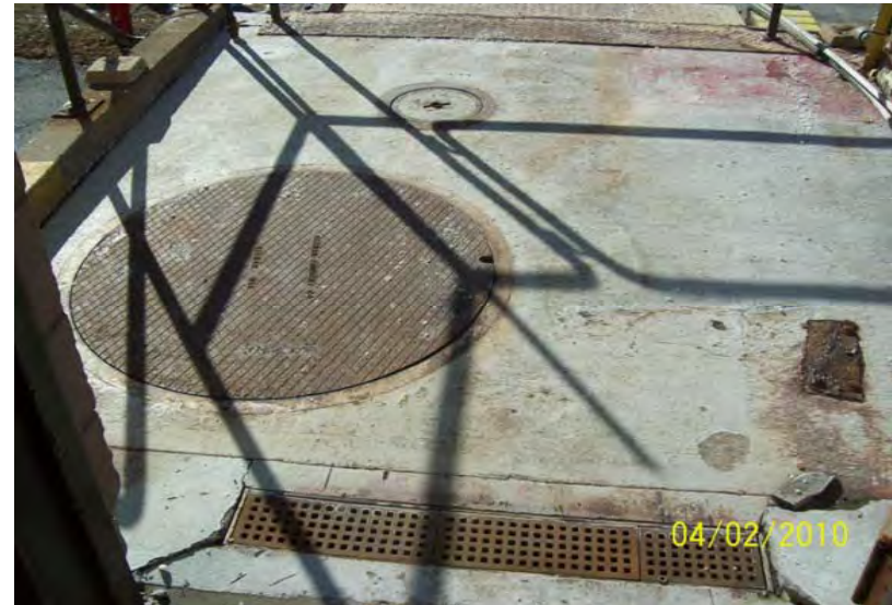
Manhole to access Tank 208 and clean out port to pump out Tank 208.
