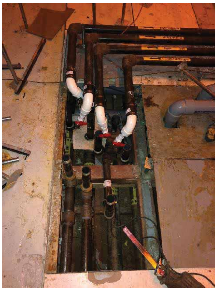
Solvent Pipe Pre-Removal
