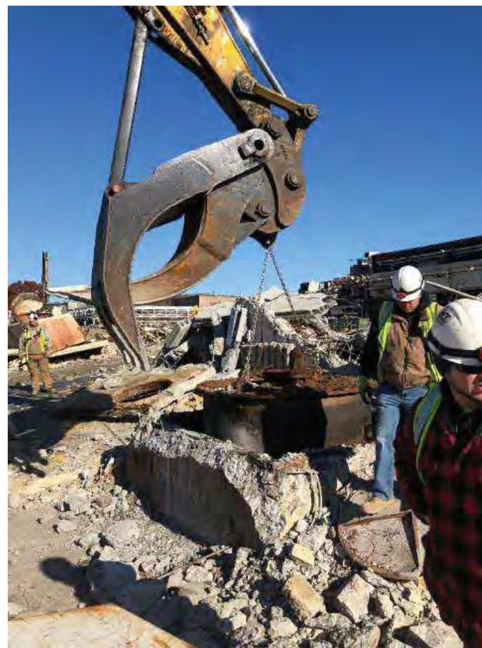
Removal Of Previously Closed Out Solvent Tank
