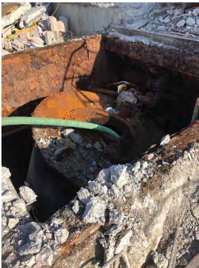
Pumping Water Out Of Solvent Tank
