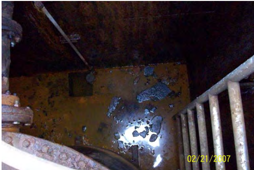
Water noted pooling within the containment dike of Tank 208.
