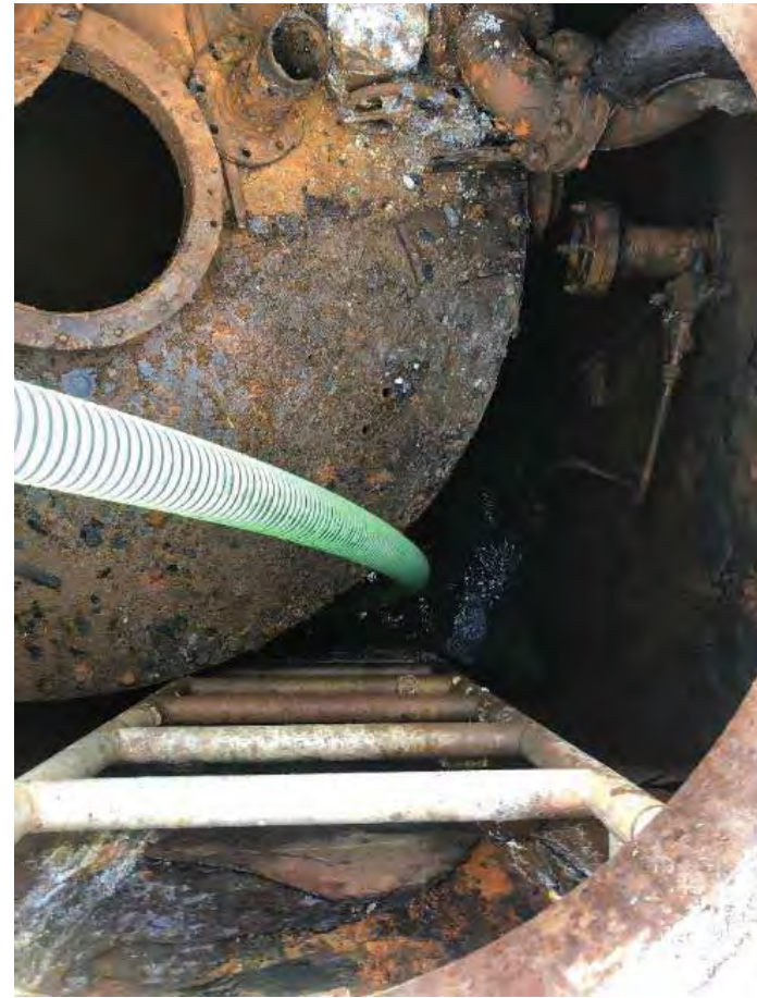
Pumping Water Out Of Solvent Tank And Vault
