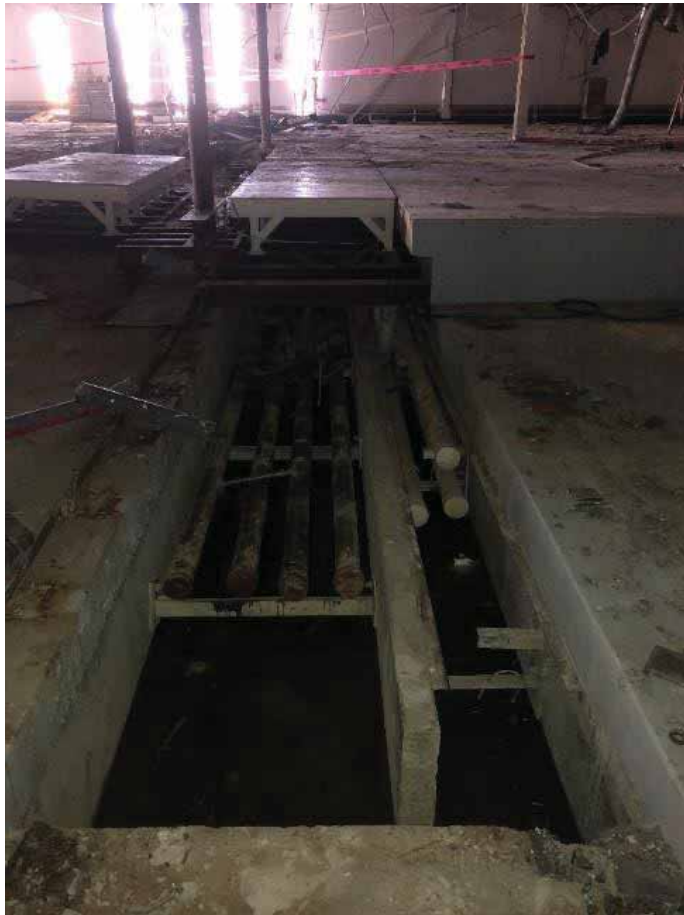
Industrial Waste Pipe Before Removal
