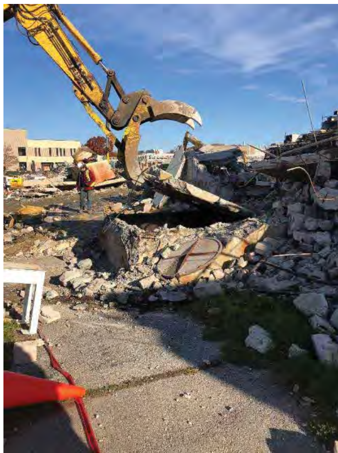
Removal To Top Of Tank Vault
