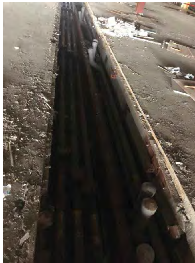
Solvent Pipe In Trench
