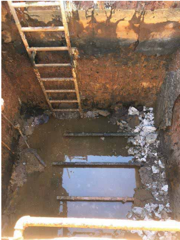
Inside Vault After Solvent Tank Was Removed
