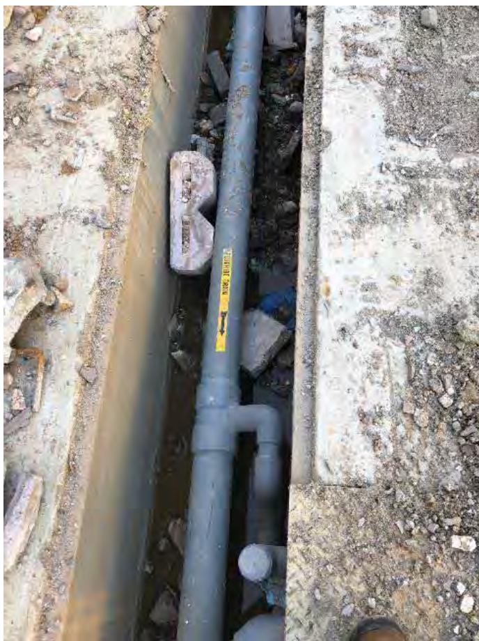
Fluoride Pipe Pre-Removal
