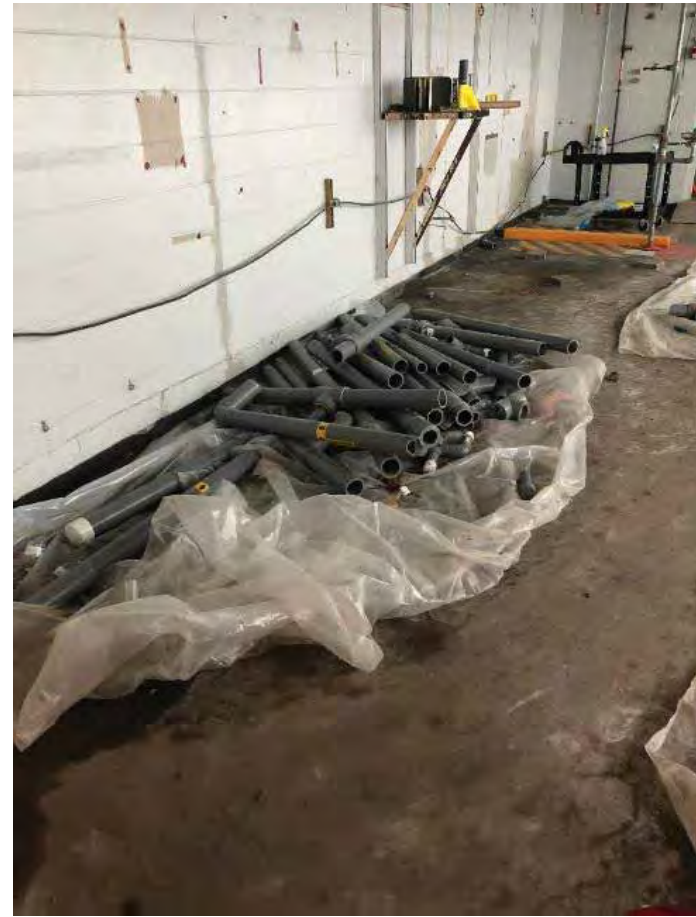
Fluoride Pipe That Has Been Removed From B322 Waiting To Be Cleaned
