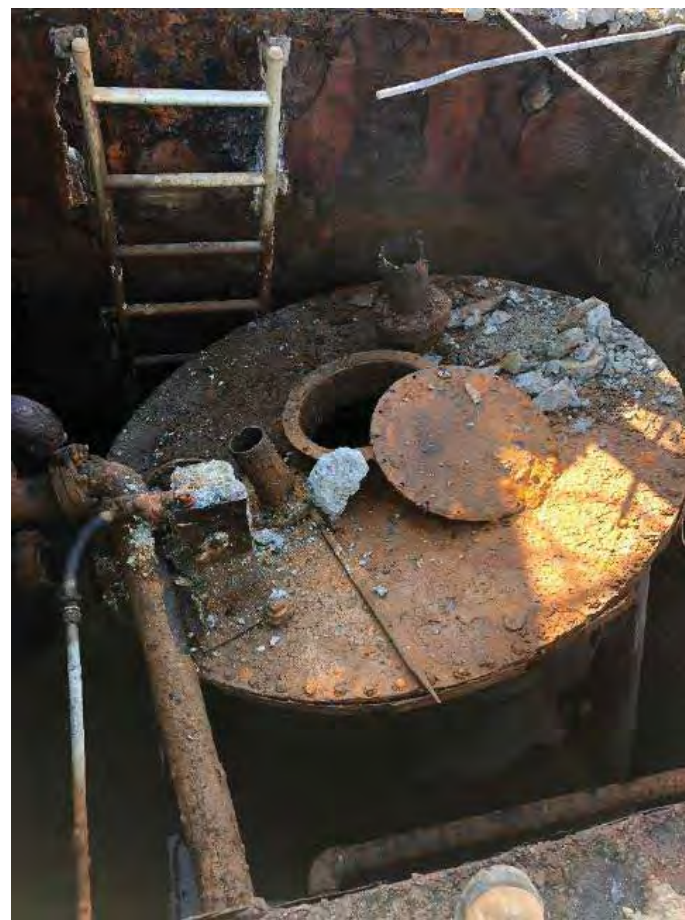
Solvent Tank Inside Vault
