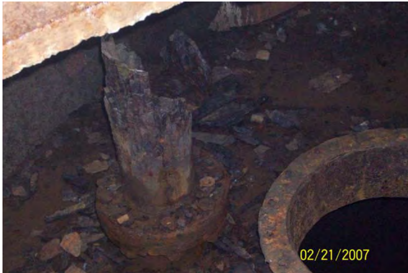
Deteriorated clean out pipe associated with Tank 208.
