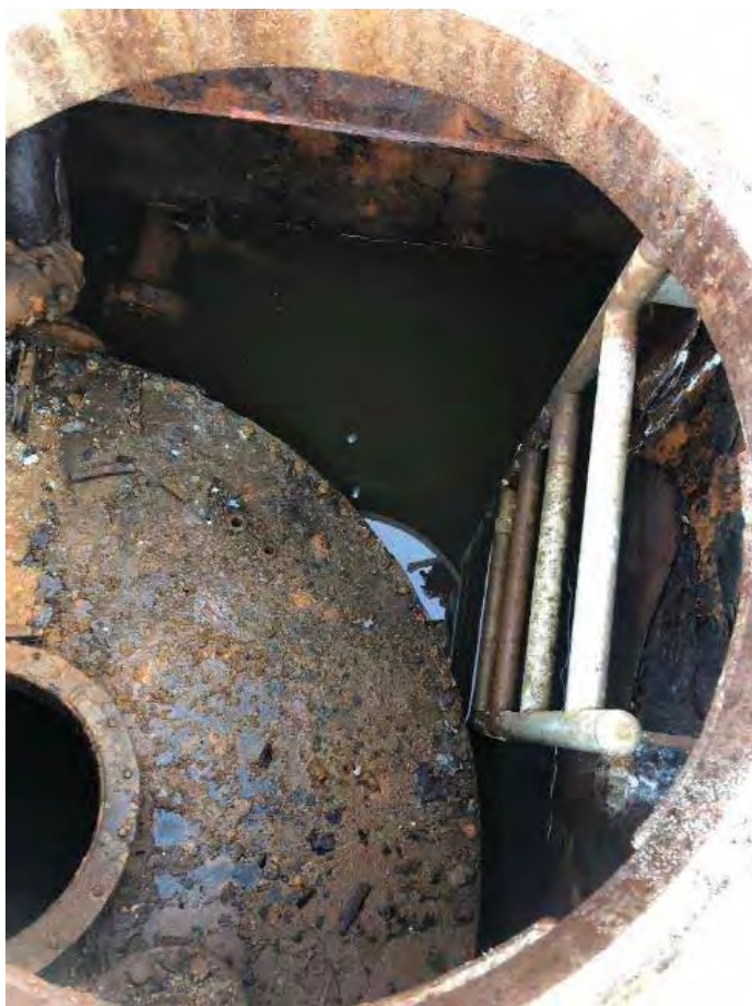
Water In Vault Prior To Being Pumped Out
