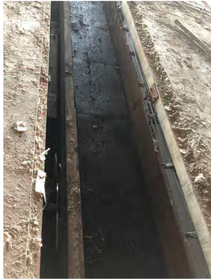
Cleaned Trench After Fluoride Pipe Was Removed
