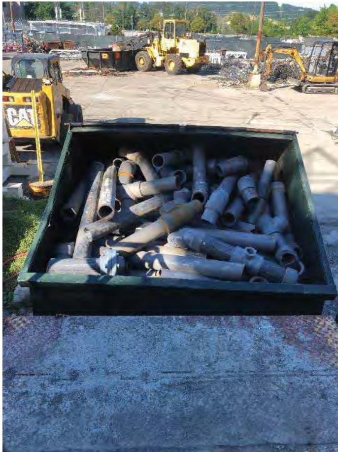
Industrial Waste Pipe Loaded Out In Dumpster After Sampled And Inspected
