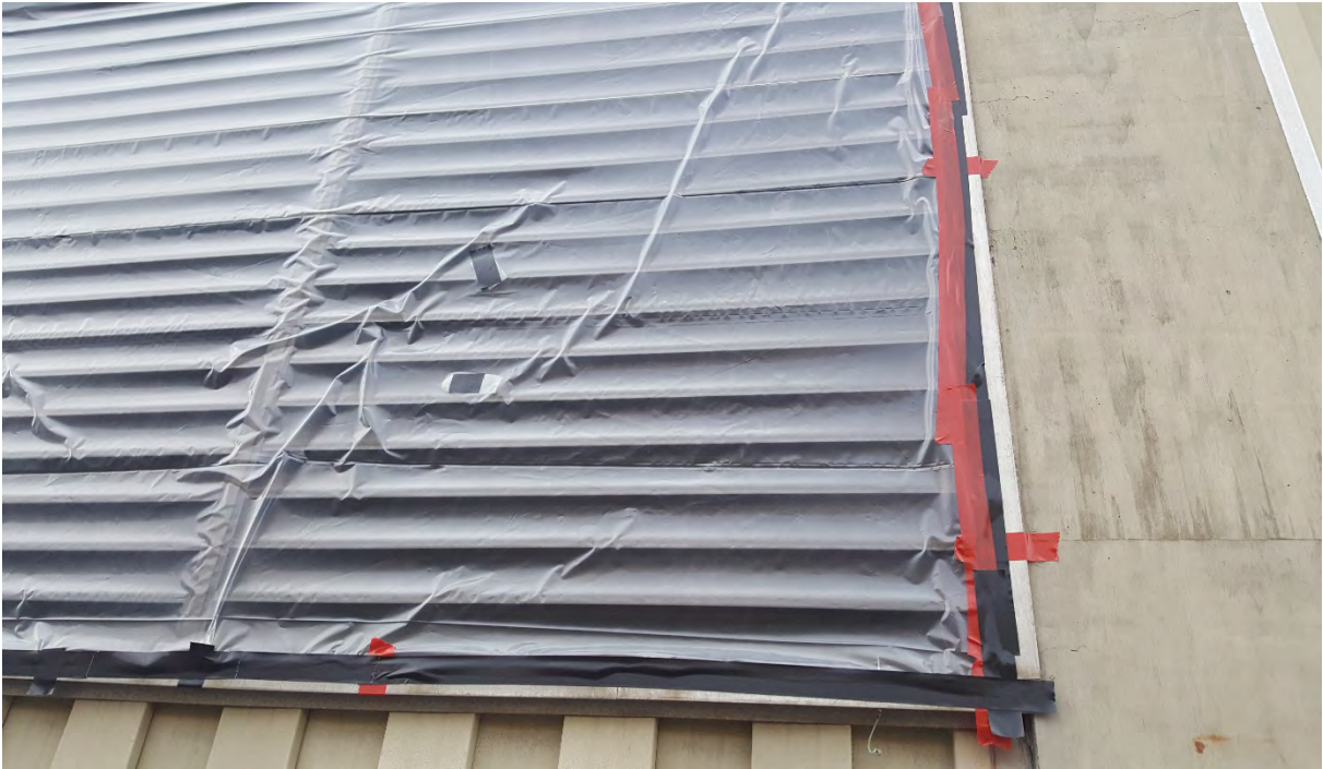
Photo 11: Close-up of air louvers covered with plastic during pressure testing
