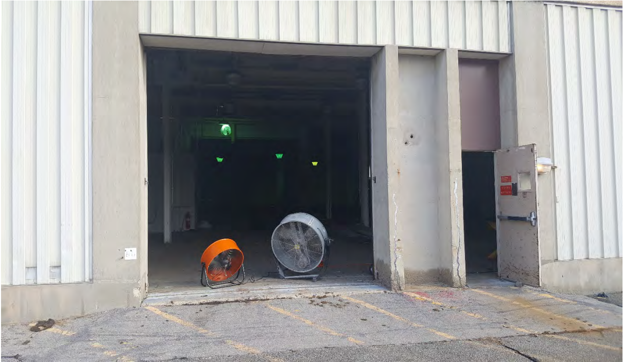
Photo 9: Fans during flush-out for pressure testing
