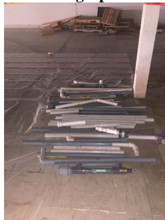
Acid SWMU Piping Post-Decontamination
