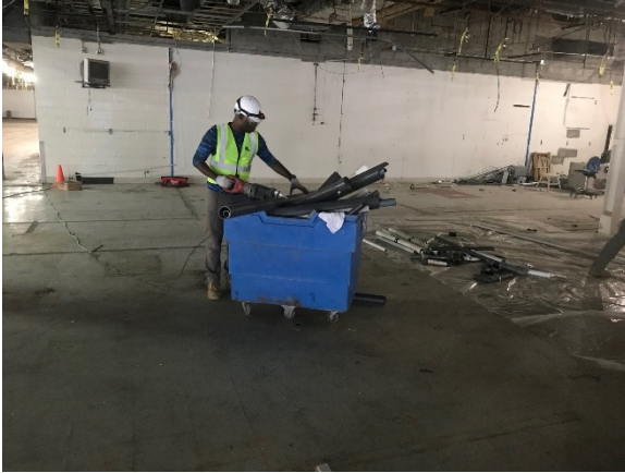
Worker Cutting Decontaminated Piping Sections for Disposal
