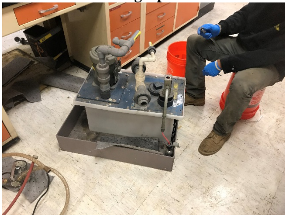
Acid Lift Station After Removal
