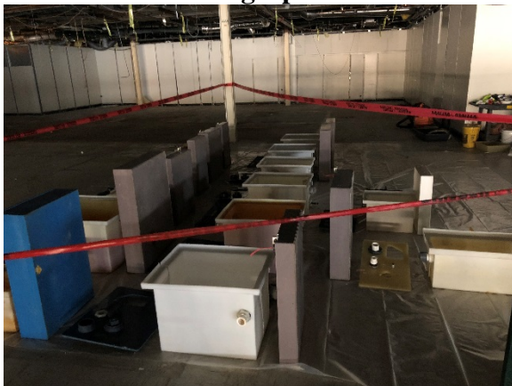
SWMU Components Post-Decontamination
