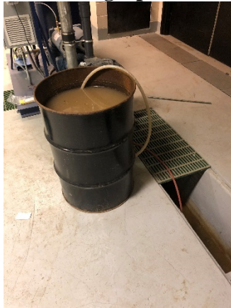
Wash Water Being Transferred From Drum Into Active Industrial Waste Lift Station
