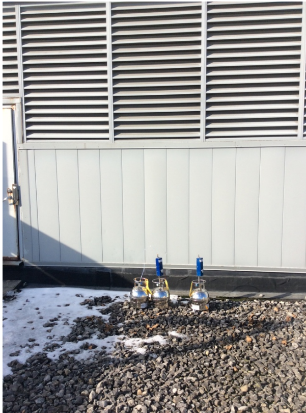
Photo 1: Samples AA0304 and FB-01; located on the roof of B386 at the intake for AHU-1.
