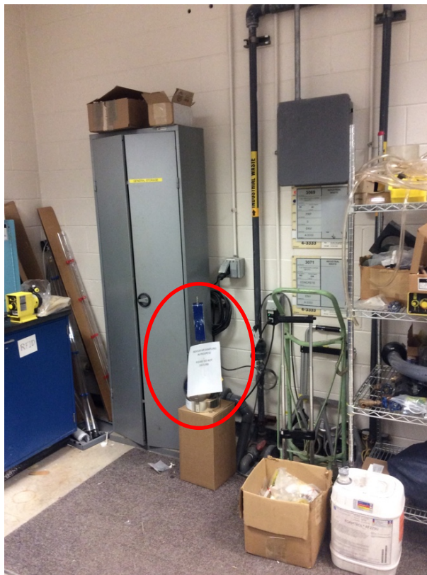
Photo 2: Sample IA0300; located in a workshop/storage area.
