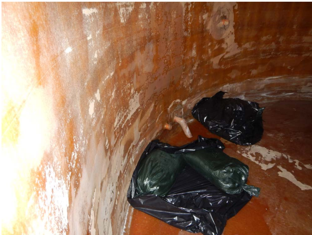
Photograph 3: SWMU 214, influent storage tank at the time of sampling on April 27, 2018.
