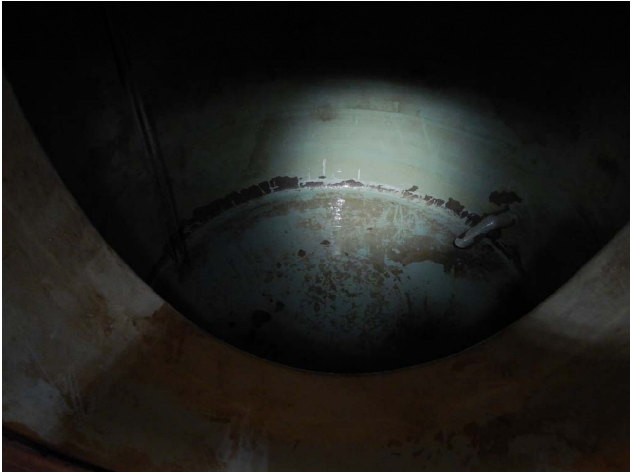
Photograph 5: SWMU 3198 air stripper effluent tank interior at the time of sampling on April 27, 2018.
