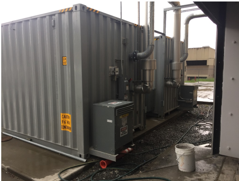
Exhibit 3.2: SSD Equipment Enclosures Exterior (System VE-7 on Left)
