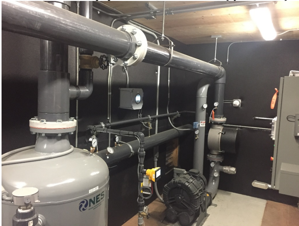
Exhibit 3.2: SSD Equipment Enclosures Exterior (System VE-7 on Left)
