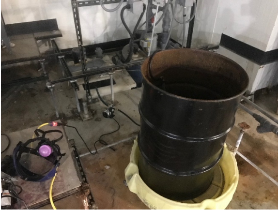
Liquids Being Transferred From Lift Station Into Drum for Later Disposal
