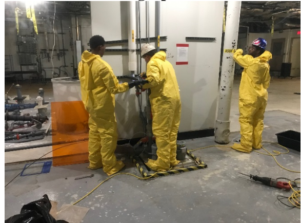
Worker Removing Supports from SWMU
