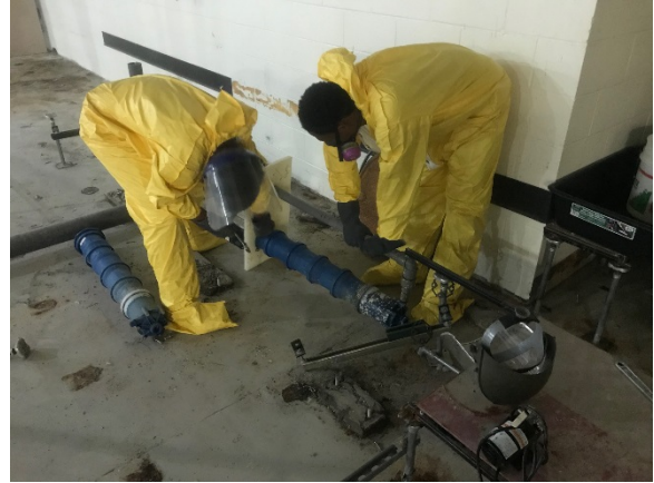
Workers Disconnecting Piping Sections
