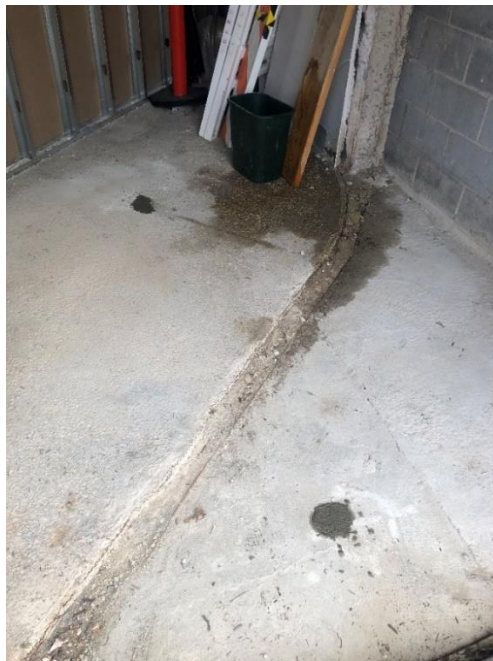
Photograph 4 Completed slab restoration.
