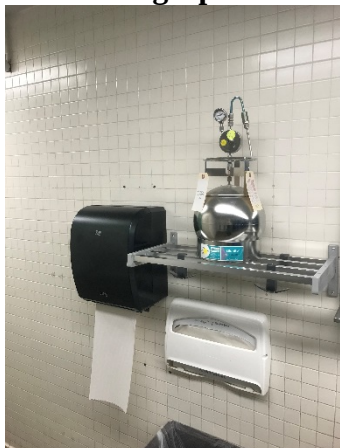
Sample Location IA-1, located in Men's Restroom
