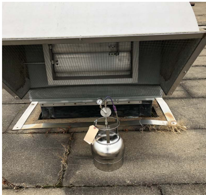
Sample Location AA-1, Rooftop
